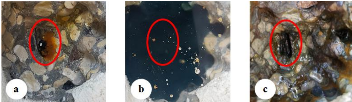
Figure 3-3 The progress of corrosion over a) 5 days, b) 7 days, and c) 49 days
