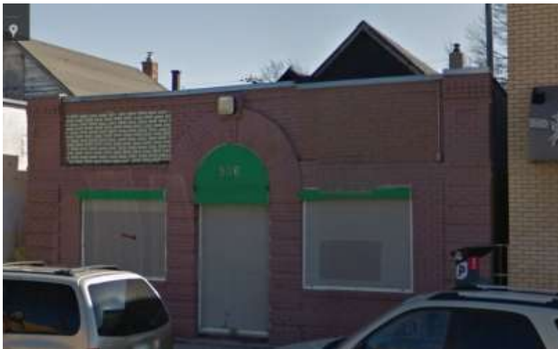
Fig 5. Small storefront on Selkirk Ave. Photo by Google Maps (2012).
