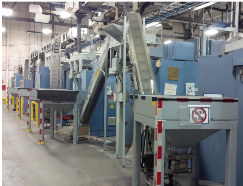
Figure 43. F-line coining presses and conveyance systems [6].
