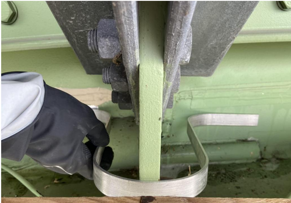
Figure 7.3: Pi-bracket over a vertical stiffener
