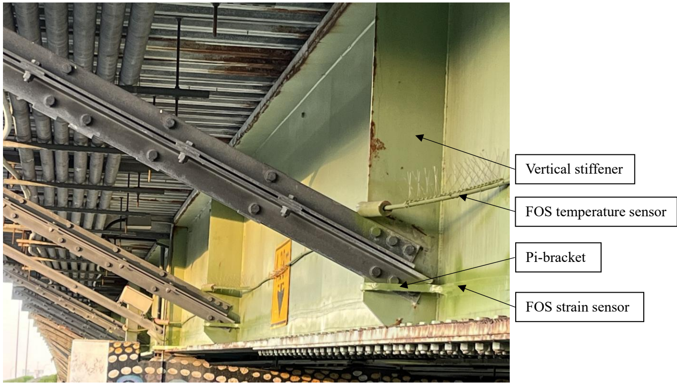
Figure 7.5: A girder of the bridge showing installed sensors
