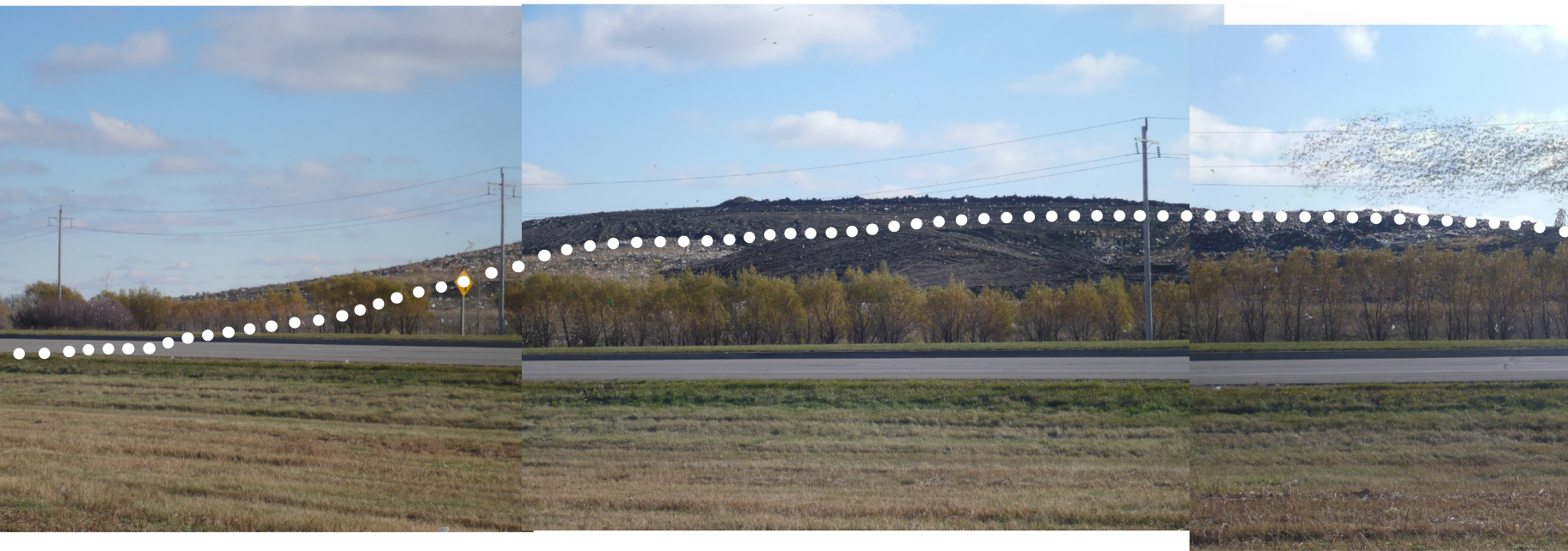
Figure 6.46 Avian Haze + Dump Topography, Brady Road Landfill
