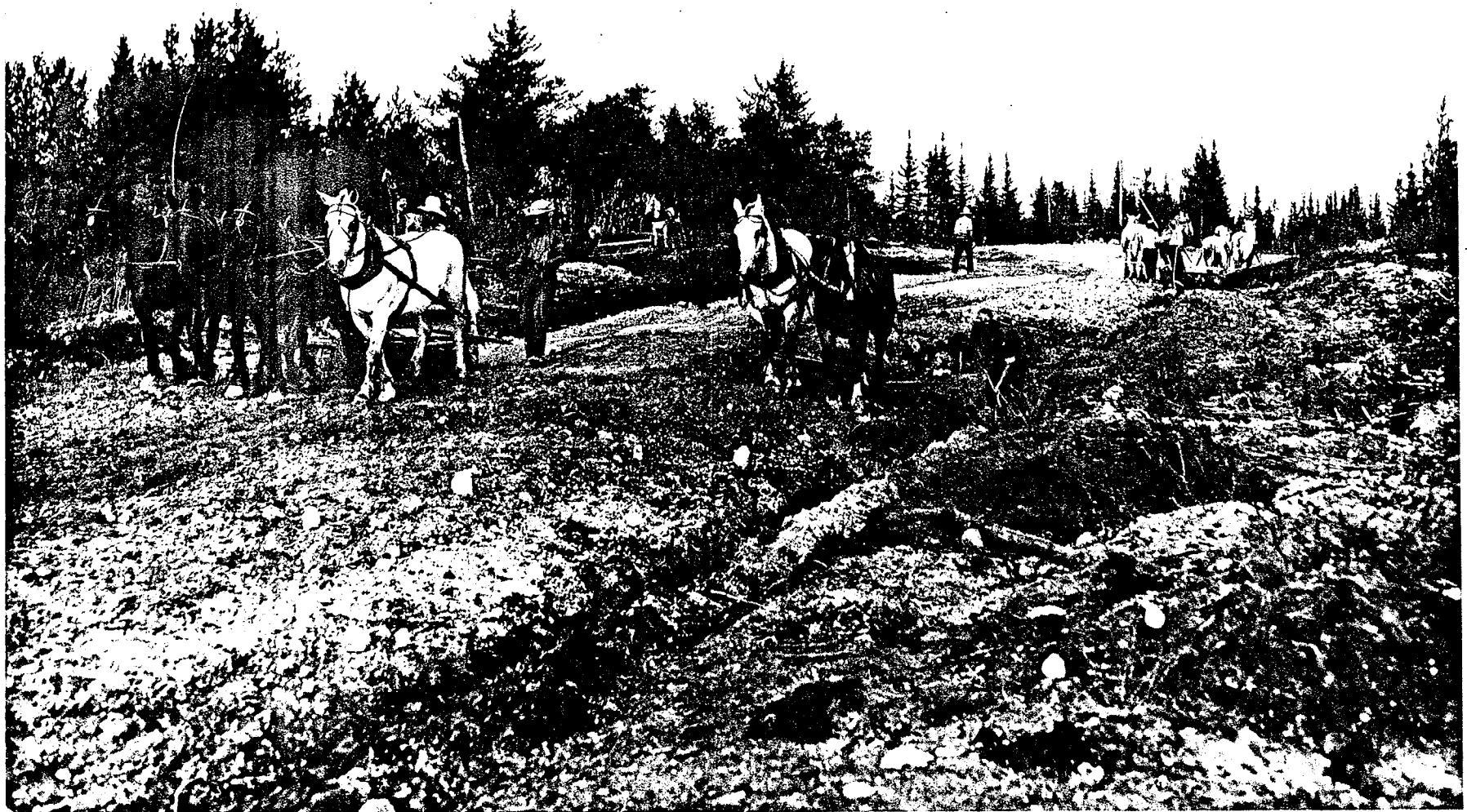
Figure 6. Road Construction Crew, (c. 1930) (Courtesy of Riding Mountain National Park)
