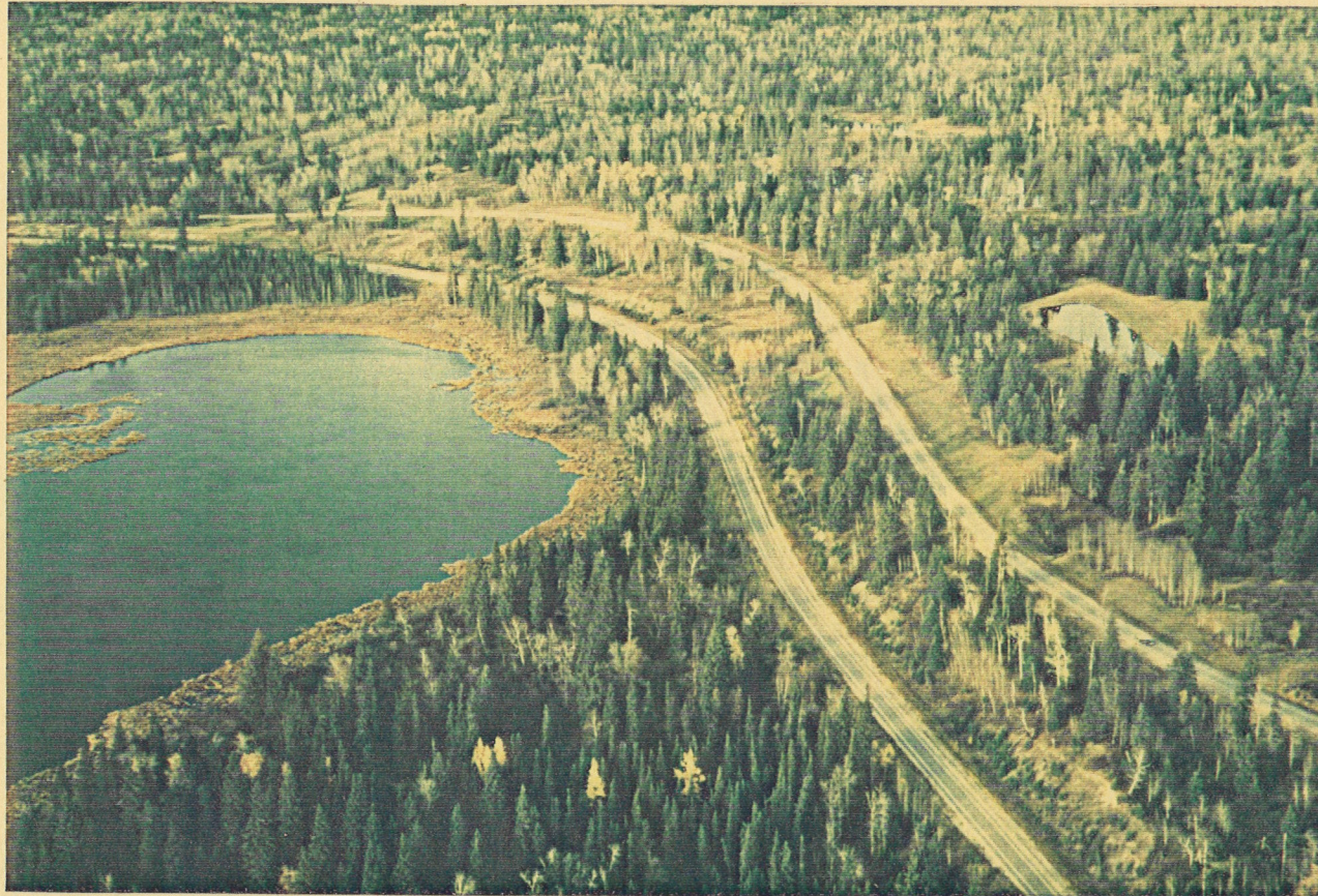
Figure 5. Aerial View of the Riding Mountain Parkway, mile 20.5
