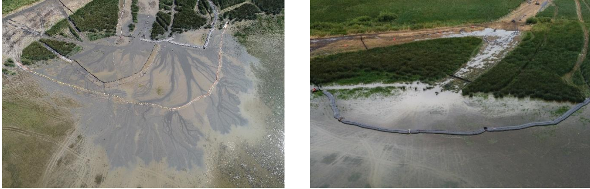
Figure 5-5 - Deltaic formation in deposition area (left) and example monitoring locations in deposition area (right)
