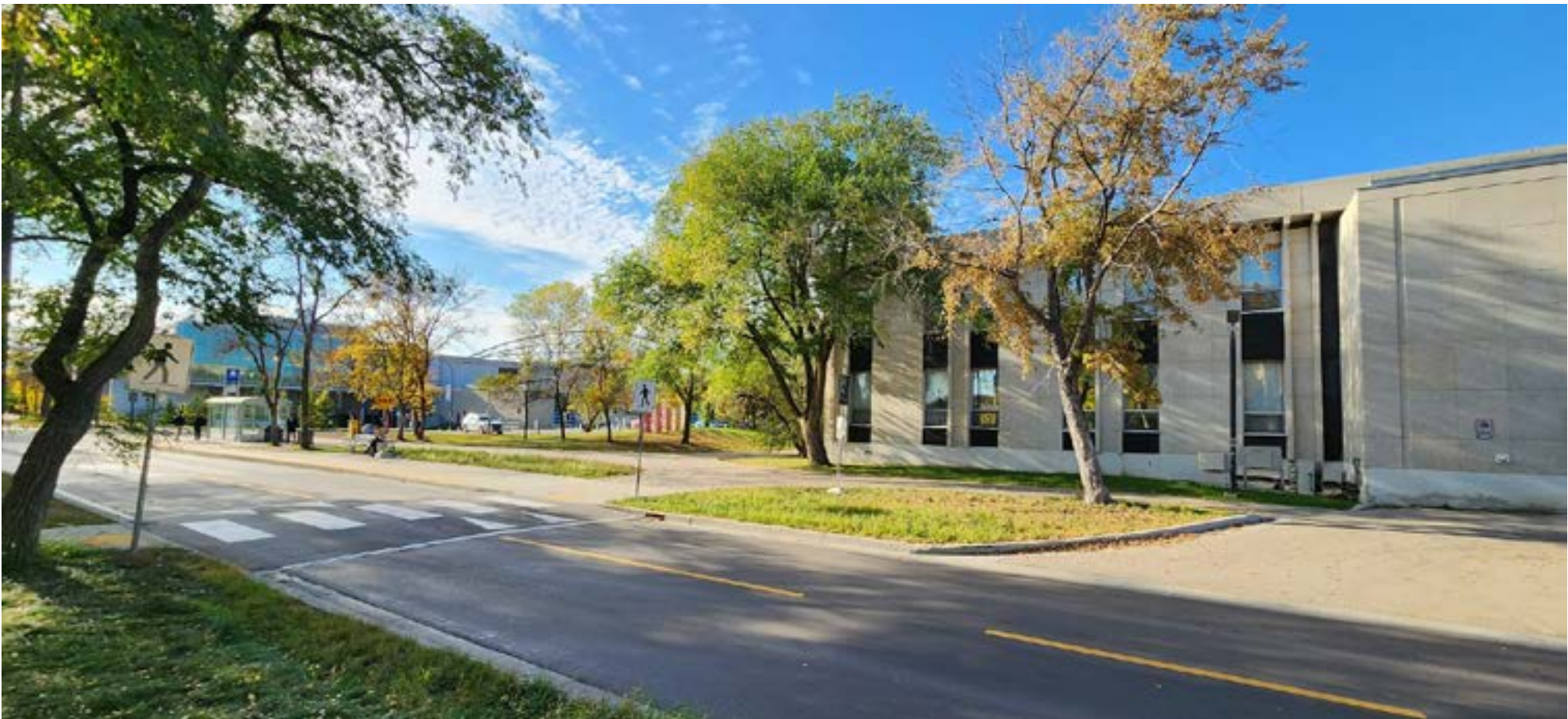
FIGURE 47: EXTERIOR FACADE - DIGITAL PICTURE - BILAL KHAN
