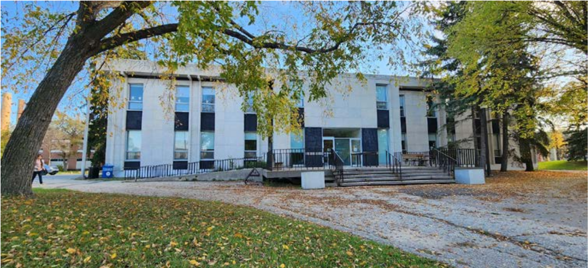
FIGURE 48: EXTERIOR FACADE - DIGITAL PICTURE - BILAL KHAN
