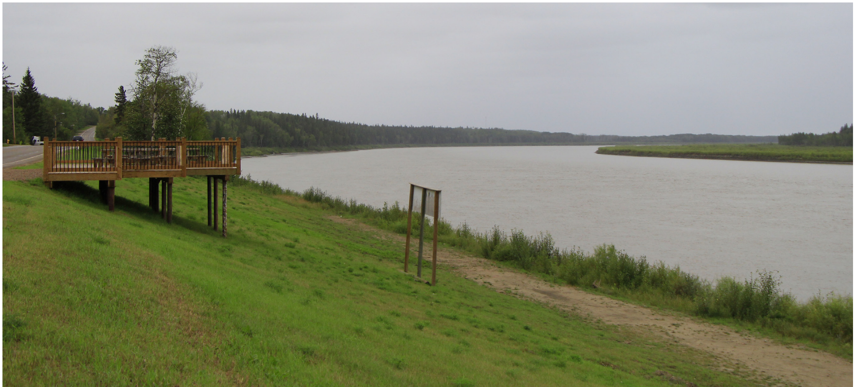
Figure 5-12: Fort Vermilion, existing Peace River access.
