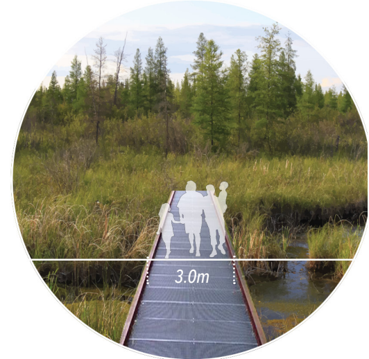
Developed Trail - Metal Grate Walkway
