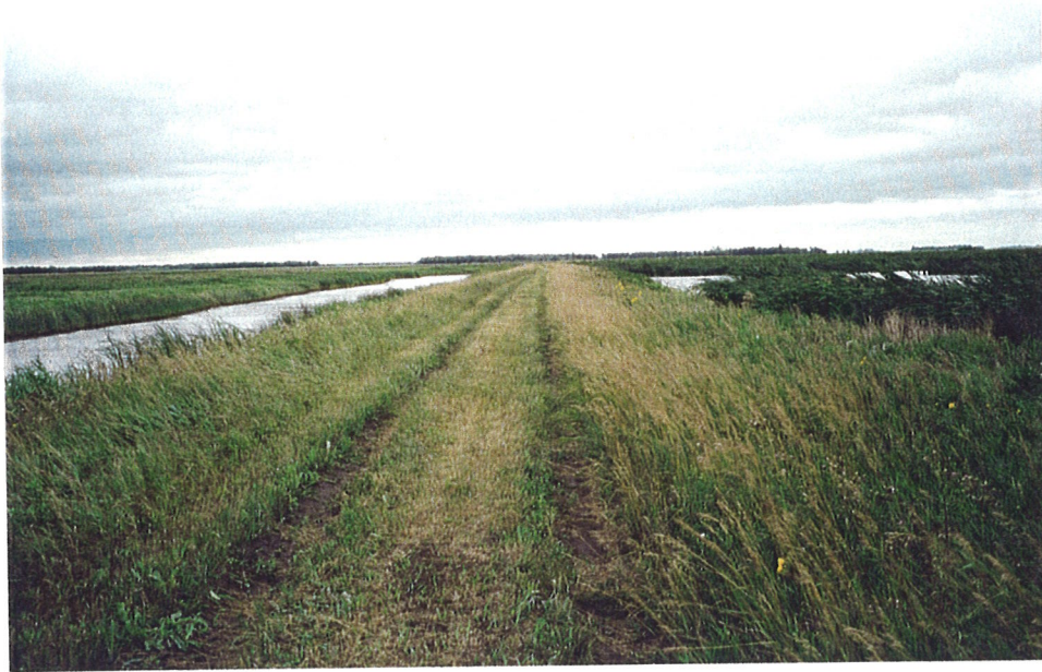
Figure 2.2. Dikes at a Ducks Unlimited Project site are constructed to be used as access trails and withstand the influence of wind and erosion.
