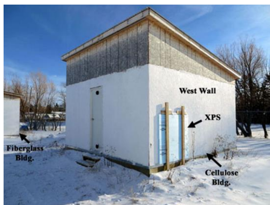
Figure 3-2: Dense pack cellulose insulation test building
