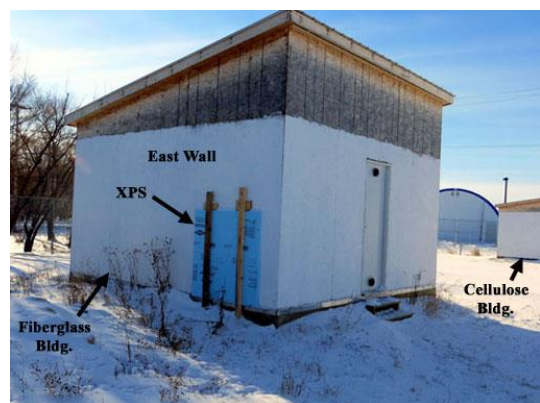
Figure 3-1: Fiberglass batt insulation test building
