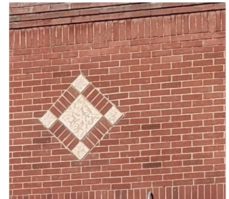
Fig. 17. Site Existing Condition [Photographs by Author]
