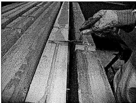
Figure 3.17: Smoothing out epoxy resin
