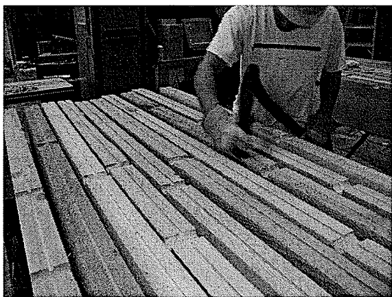
Figure 3.14: Cleaning grooves with vacuum
