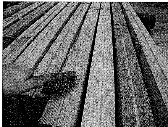
Figure 3.13: Removing loose material with brush
