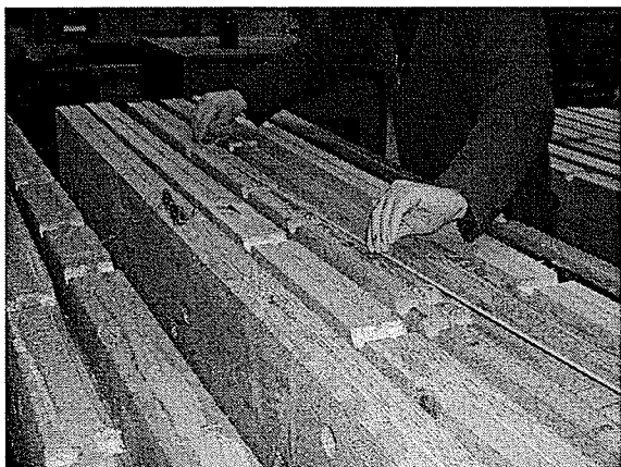
Figure 3.16: Inserting GFRP rods into epoxy-filled grooves
