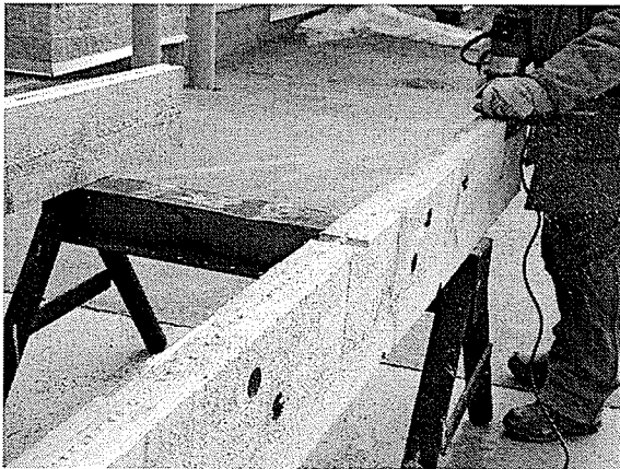
Figure 3.12: Routing grooves along bottom of beam
