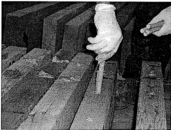
Figure 3.21: Inserting GFRP rods into epoxy-filled grooves
