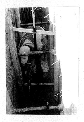
View showing vertical movement gauges and placing of sand back-fill at Clifton Street installation.
