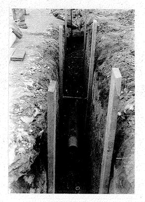
View showing trench, shoring and vertical pipe movement gauge in background. Richard Avenue installation.
