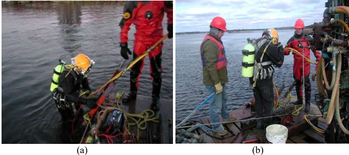
Figure 24: Surface-supplied tethered diver entering water to perform final cut-off of drill rods and install connecting plate and nuts. Back-up diver (red suit) provides assistance and is geared-up for quick response.
