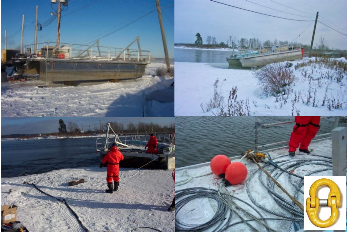
Figure 26: Clockwise from top left: Pontoon test platform assembled on shore. Vessel on snow ramp with front of pontoons digging into surface ice. 32 mm (1-1/4”) main mooring cables (underfoot) and typical marker buoys on deck of vessel. At point ‘A’ after maneuvering across the bay to the north and west of the main anchor points. Inset: hammerlock style connection for main cable to the chain main link.
