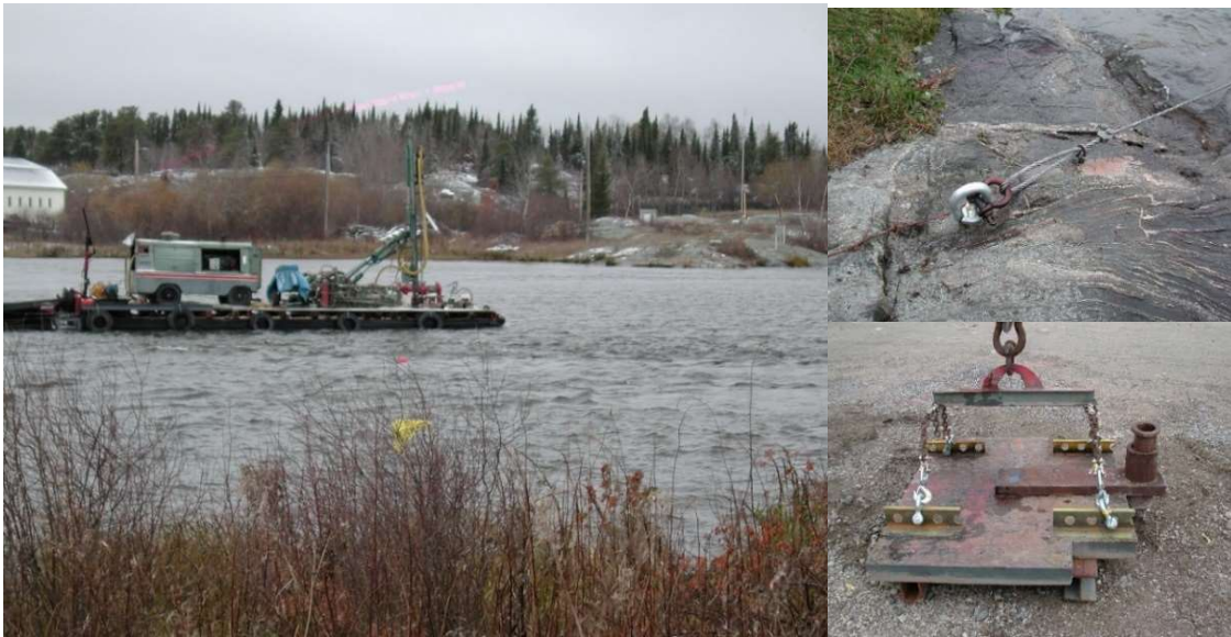
Figure 21: Clockwise from left: (a) barge in place at drilling location 2, buoy marker in water and yellow marker on shore provide alignment, (b) rock anchor on shore for 9.5 mm (3/8") positioning cable from winch on the barge, and (c) the drill plate on shore showing collar for drill pipe on right and lowering brace with adjustable balance points.
