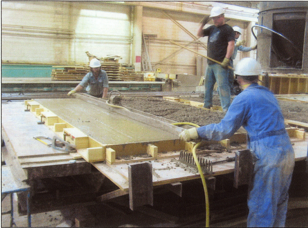
Figure 4-4. Compaction of Concrete using Vibratory Concrete Screed.
