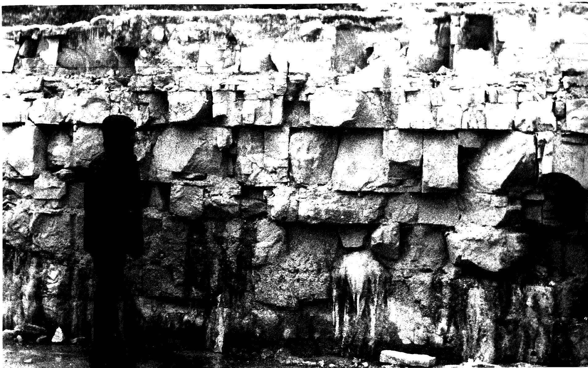
Fig. 10. Upper bedrock zone under the Red River Floodway Inlet control structure.
