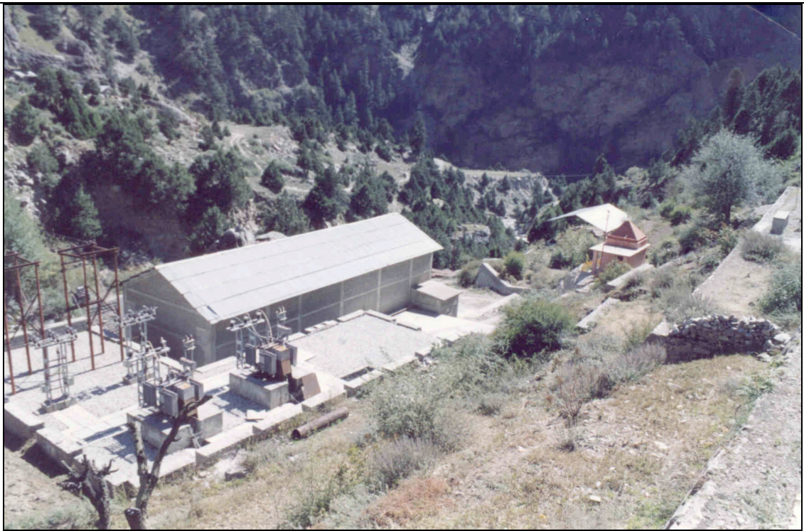
Plate 4-11: Jumma hydro plant.
