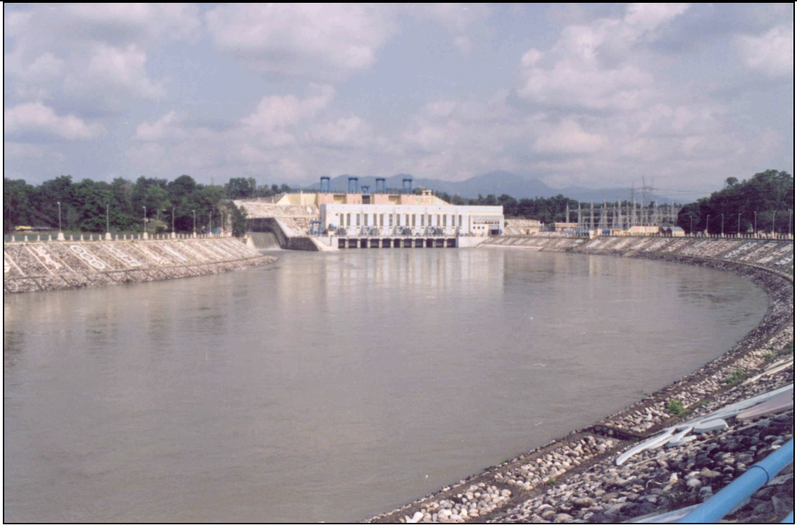
Plate 2-1: The Chilla Dam on the Ganges near the City of Haridwar in Uttaranchal.
