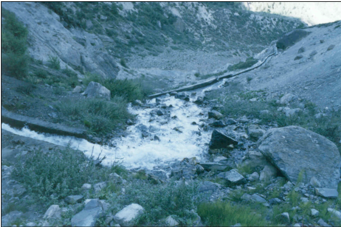
Plate 4-2: Malari Hydro Station diversion channel.
