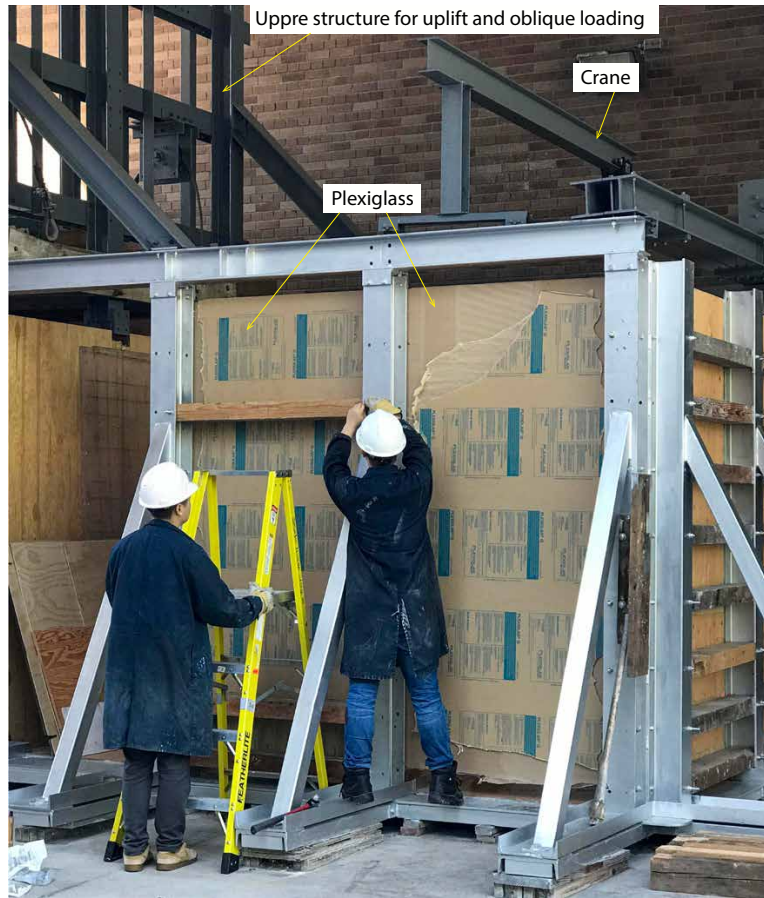
FIGURE C.1: Test preparation: plexiglass installation
