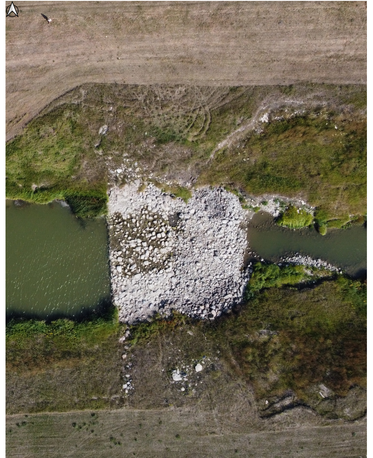
Fig 75. Drone aerial showing different channel widths by rock outcropping transition, Jul 2023
