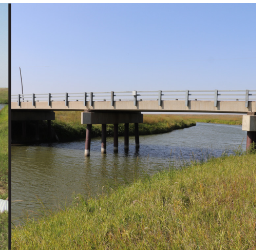
Fig 82. Another bridge variation on the Norquay Channel, Jul 2023
