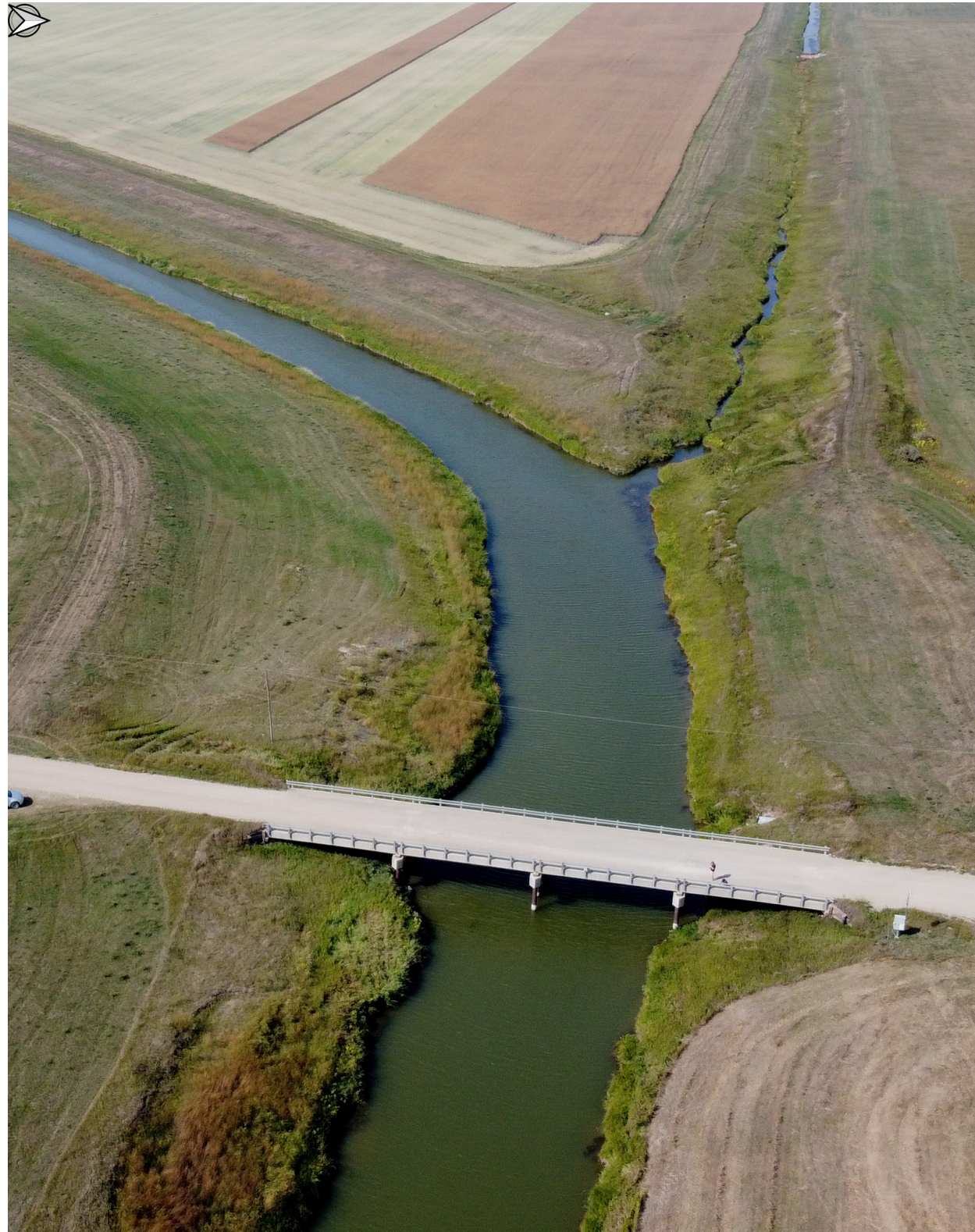
Fig 76. Drone aerial showing the channel convergence of the Carrother's Drain, Sep 2023
