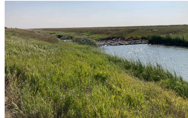
Fig 77. Water level difference at rock outcropping on the Norquay Channel, Jul 2023
