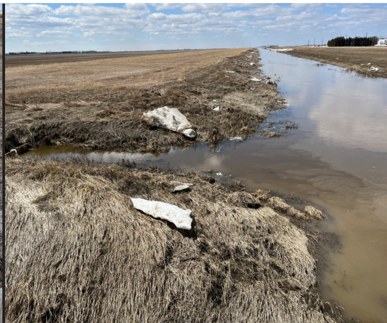
Fig 57. Culvert outlet with dark field runoff on the Norquay Channel, April 2023
