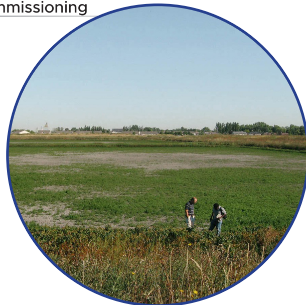
Fig 92. Decommissioned lagoon cell in Niverville
