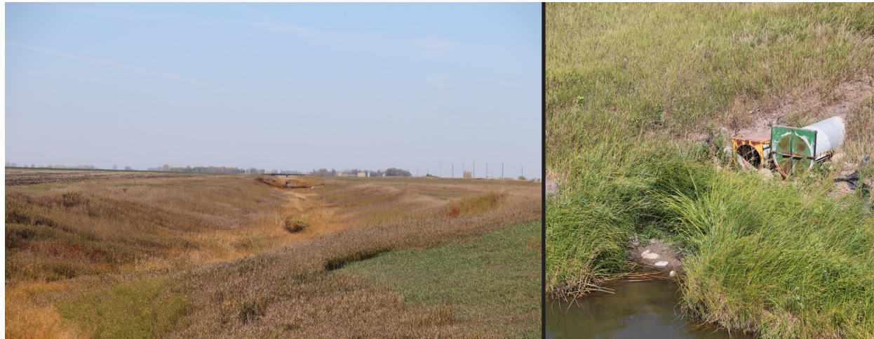
Fig 69. View of Carrother's Drain facing west with vegetation, Sep 2023
