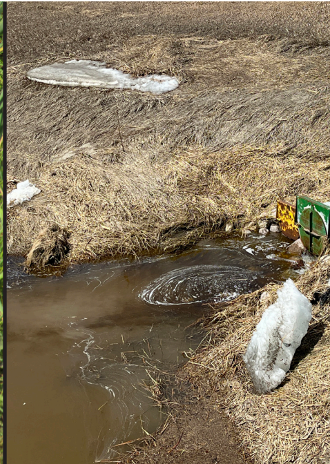
Fig 55. Culvert outlet on the Norquay Channel, April 2023
