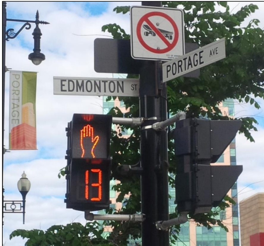
Figure 4 Pedestrian Countdown Housing Configuration
