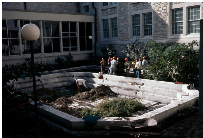
Fig 6.1.2 Photos during construction, n.d.
