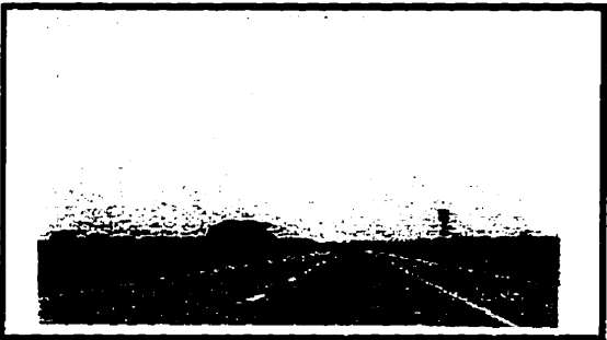
[11] Southbound direction--just north of Water Town, South Dakota
