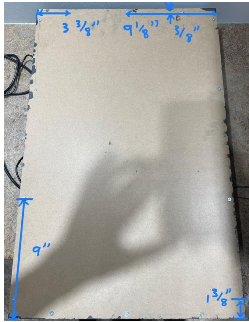
Figure 30. Installation of the MDF backboard
