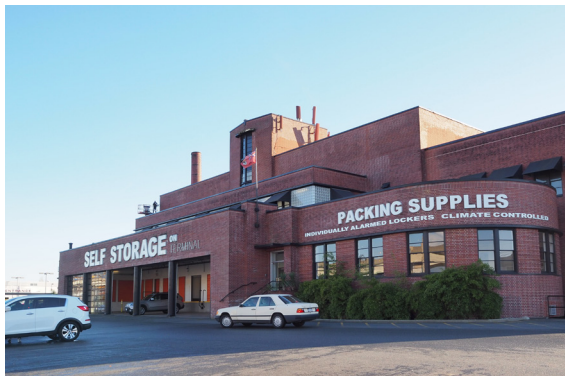
Figure 4.1-4 Canada Packers building on Terminal Avenue
