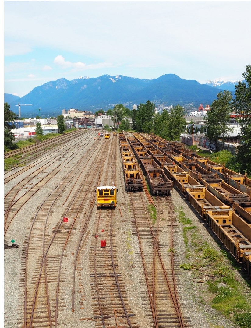
Figure 1.1-9 Rail yards in False Creek Flats
