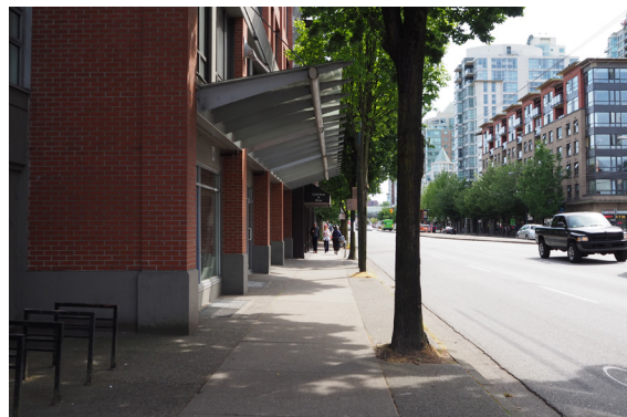
Figure 4.1-20 Main Street looking south
