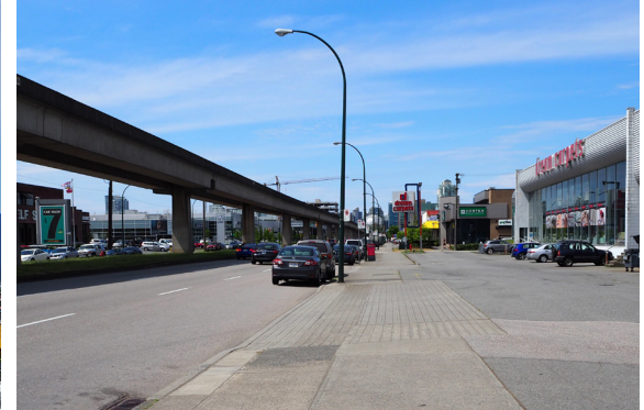
Figure 4.1-41 West on the north side of Terminal Avenue
