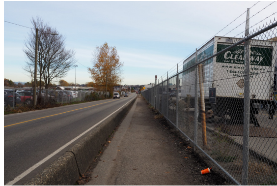
Figure 4.1-22 Pathway on National Avenue facing east
