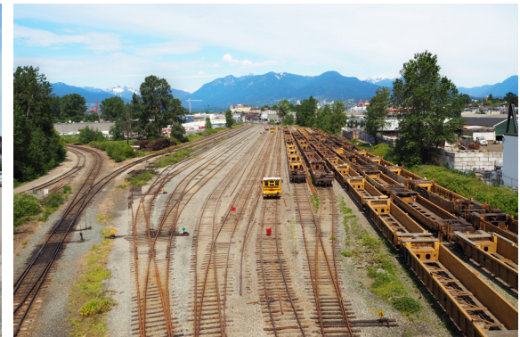
Figure 4.1-17 Rail yards north of the Grandview Viaduct
