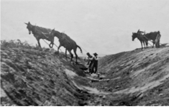
Figure 4.3. (above) 6' drainage ditch. Adapted from "A 6' drain, N23022, 1911" from Manitoba Archives. © Manitoba Archives. Adopted with permission.
