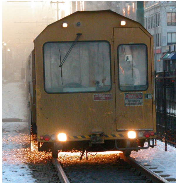
Figure 1.2: Grinding car correcting rail corrugation. The sparks flying off are from the stones grinding on the metal rails.
