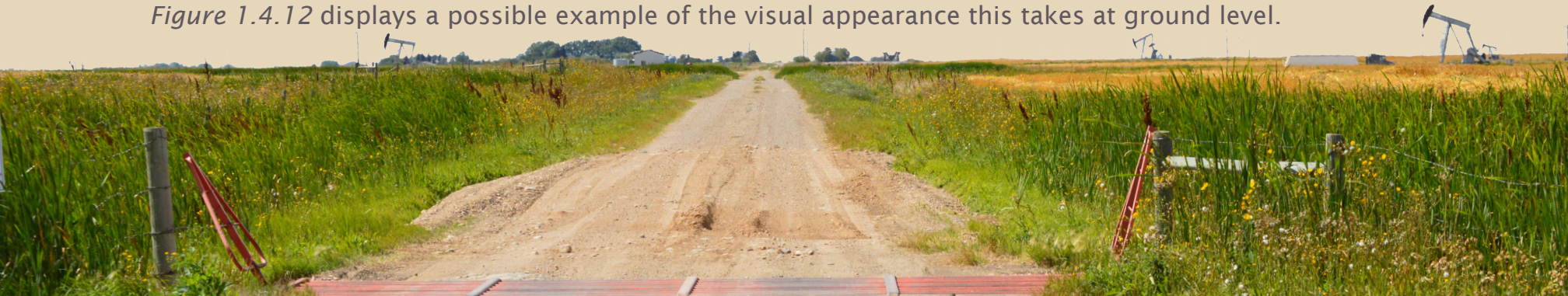
Figure 1.4.12: example of an access road at a higher elevation than the surrounding, lower conditions
