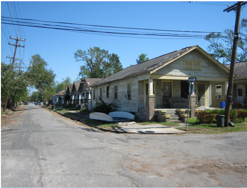
Figure 63: Uptown New Orleans row of houses with roofs damaged by Hurricane Katrina. Photo by Infrogmation. Available at http://commons.wikimedia.org/wiki/File:LowerlineBlockBack.jpg under the Creative Commons Attribution-Share Alike 2.5 Generic http://creativecommons.org/licenses/by-sa/2.5/deed.en . Accessed February 13, 2012.
