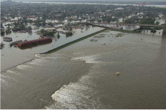
Figure 55: Aerial photograph of the break in the levee in the 9th ward. New Orleans, LA, August 30, 2005. FEMA/< Jocelyn Augustino> http://www.photolibrary.fema.gov/photolibrary/photo_details.do?id=18177 Accessed January 14, 2011. Public domain image.
