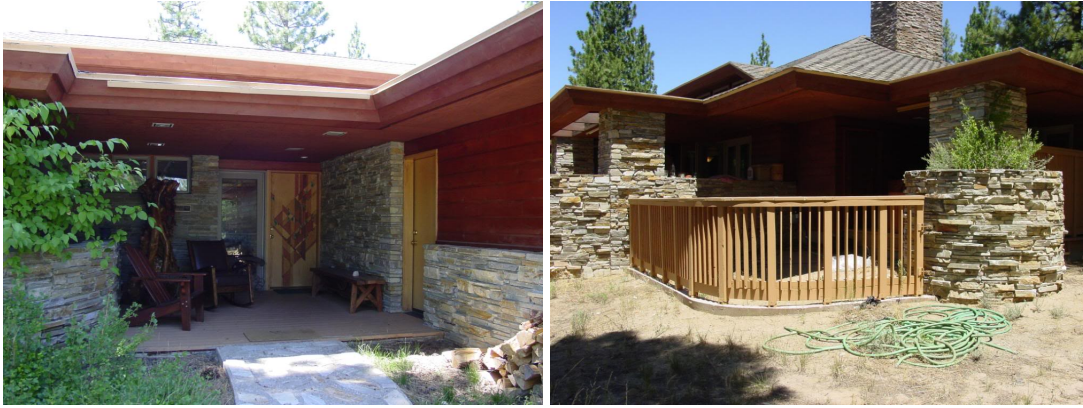
Figures 20 & 21: Covered Exterior Spaces
