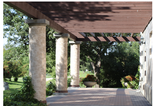
Figure 38 Assiniboine Park Pavilion pergola walkway.
