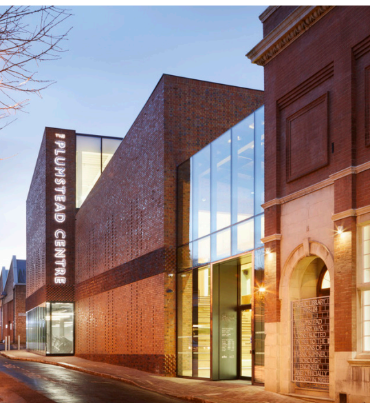
Figure 19 Plumstead Centre extension. © Jack Hobhouse
