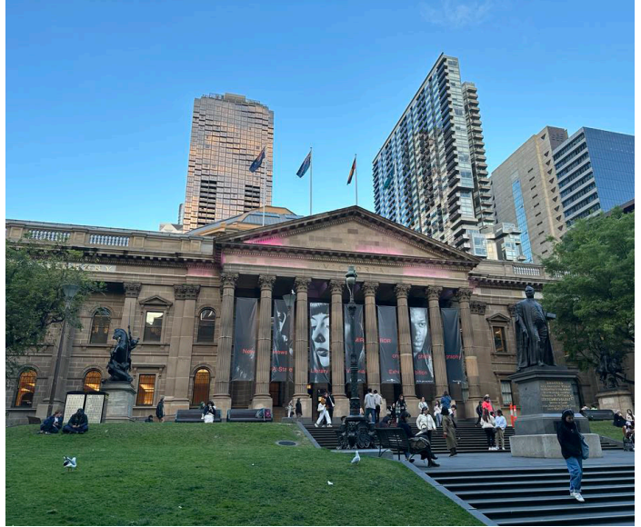
Figure 11 State Library Victoria exterior.
