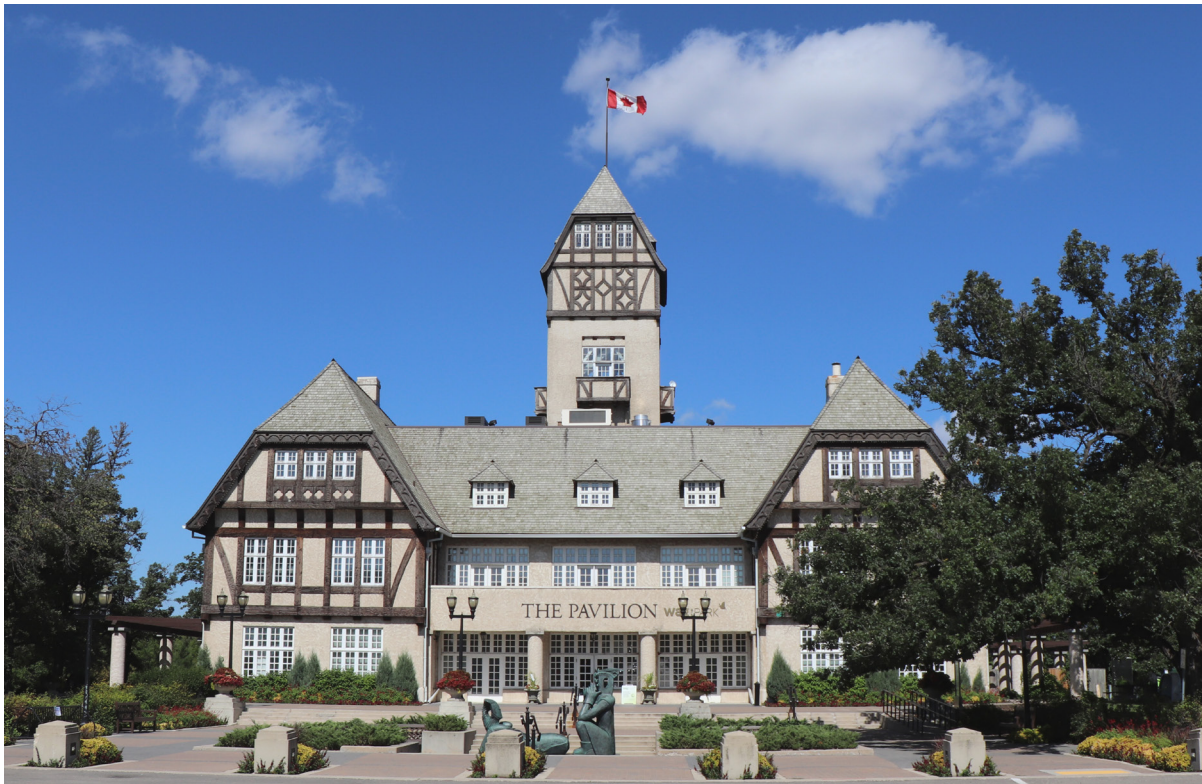
Figure 35 Assiniboine Park Pavilion south front view.
