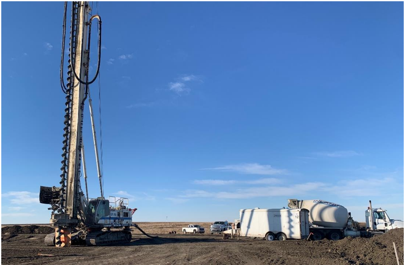
Figure 3.2. CFA piling rig featuring concrete truck and pump
