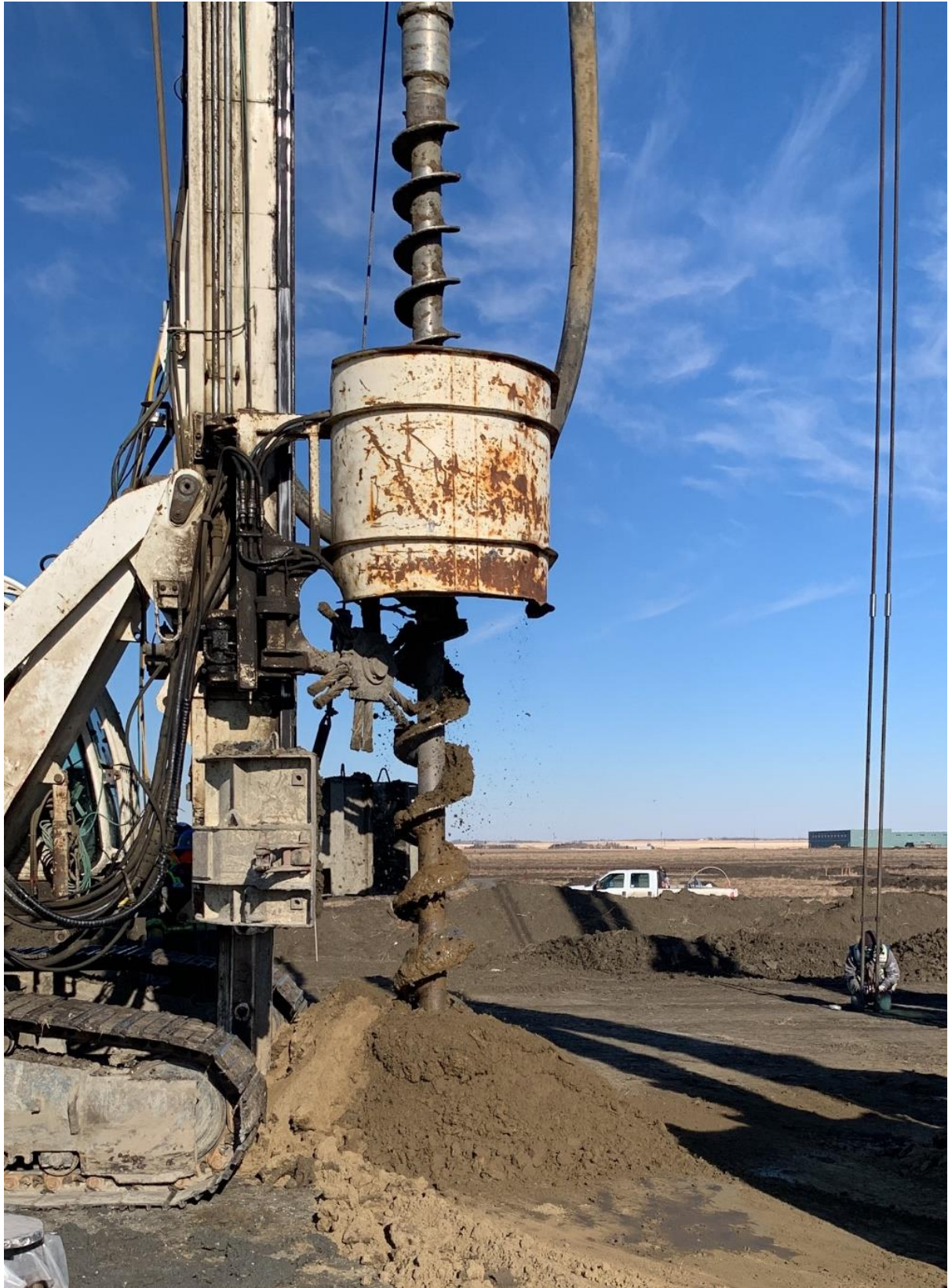
Figure 3.3 CFA piling rig during boring
