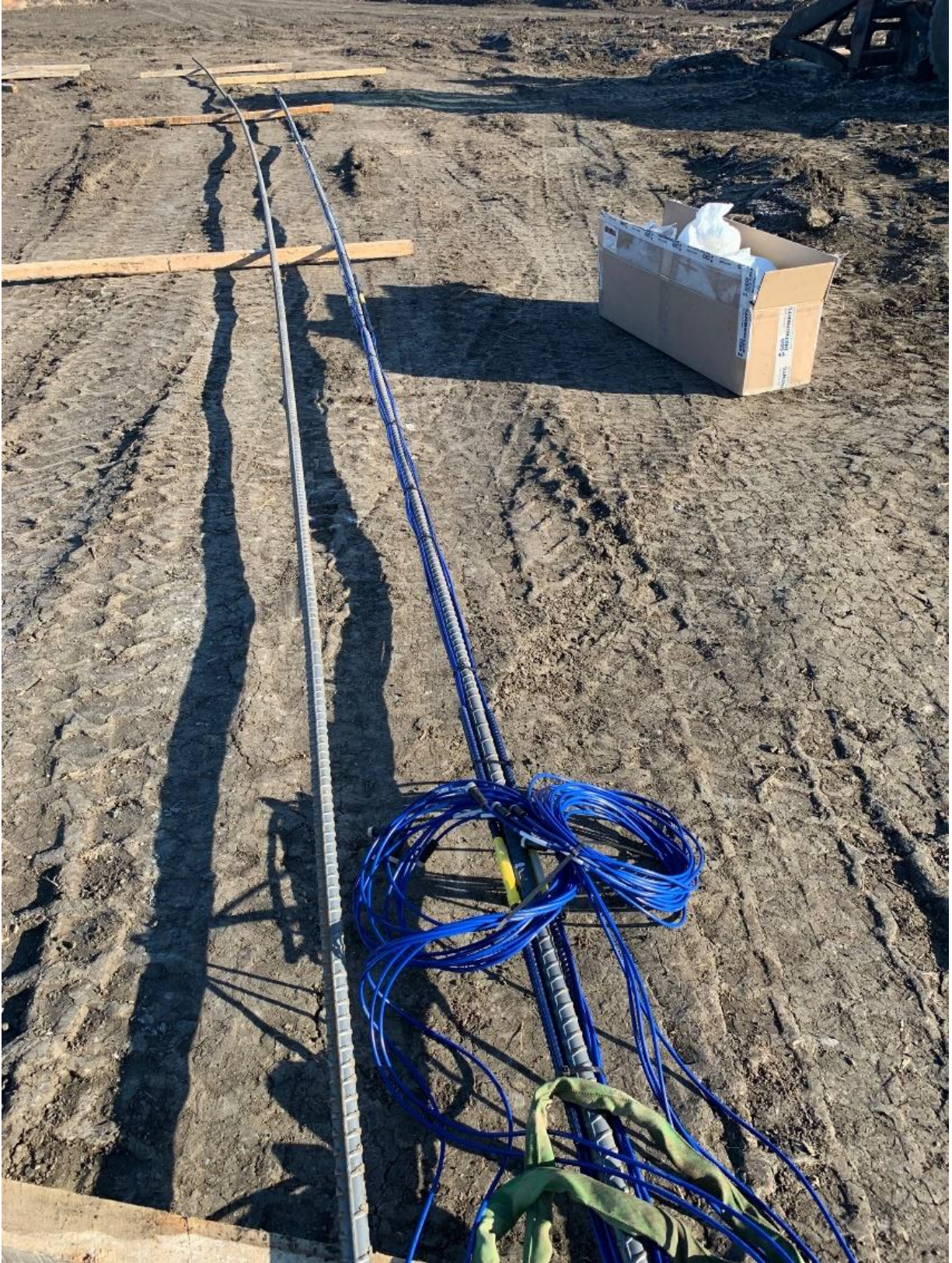
Figure 3.4. Center rebar instrumented with vibrating wire strain gauges
