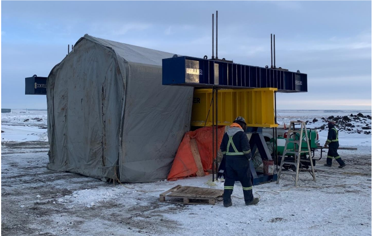
Figure 2.8. Anchor piles, load transfer beams, and test beam
