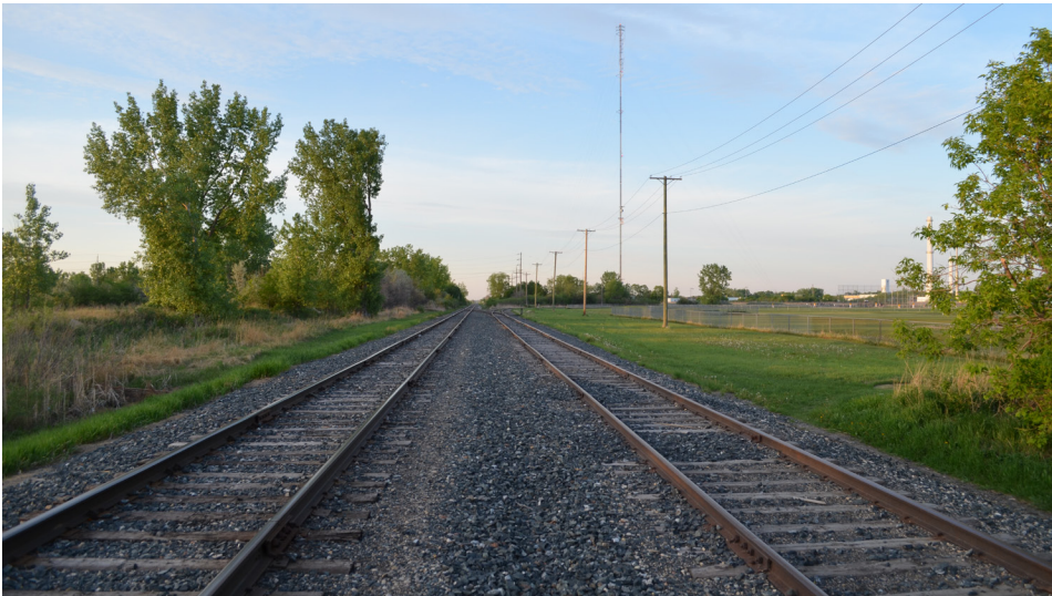
Figure 3.26 Existing Condition: Unused portion of track (right) from the Bergen Cut-Off trail that ties into the used portion of CP rail line.
