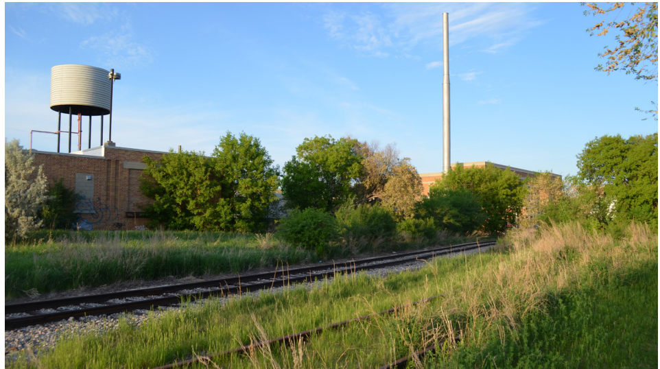
Figure 3.23 Existing Condition: Berm crosses Main St. Adjacent to the North Winnipeg water treatment facility where unused CP rail remains.
