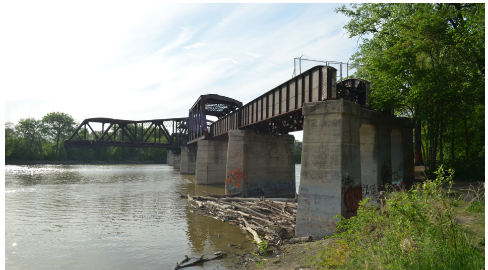
Figure 3.7 Existing Condition: Bergen Cut-Off Bridge from East Shore of Red River with Kildonan Park on the other side.
