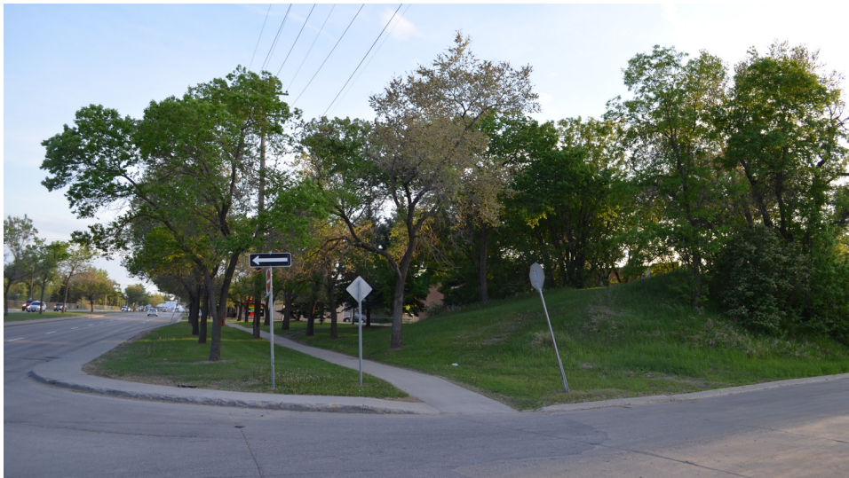
Figure 3.13 Existing Condition: Berm which supported a rail bridge crossing over Main Street by Kildonan Park Golf Course.
