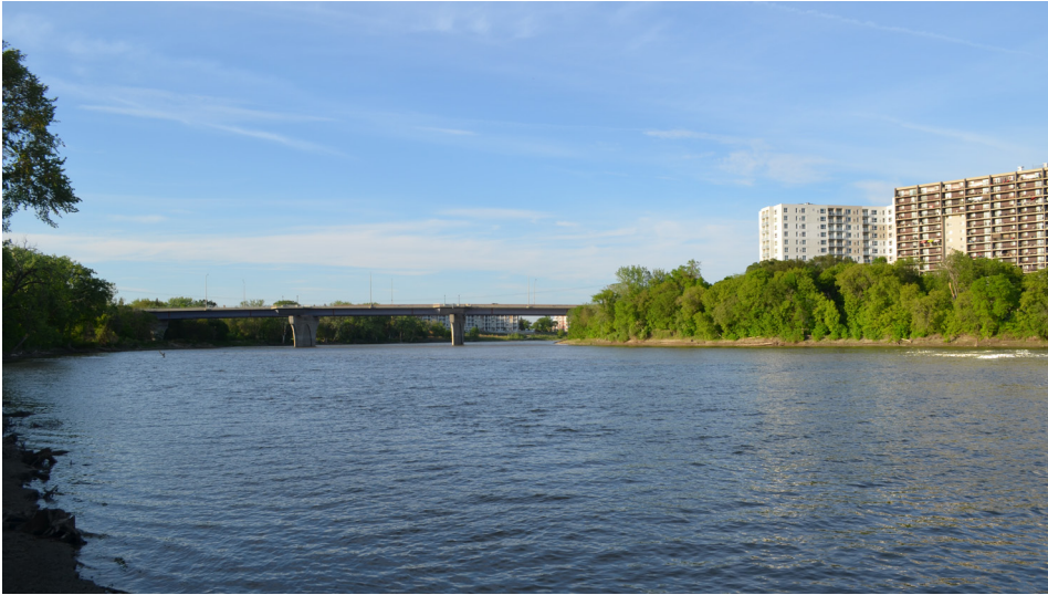
Figure 3.9 Existing Condition: Kildonan Settlers Bridge, part of Chief Peguis Trail lies in the distance from the West Shore of Kildonan Park.
