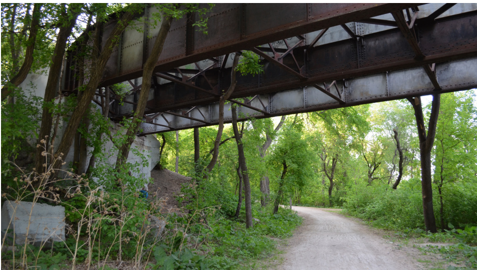
Figure 3.11 Existing Condition: Passing under the bridge along the existing trail.
