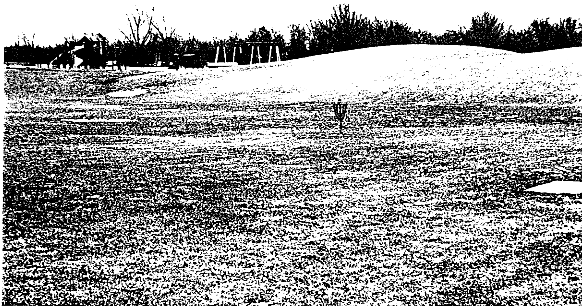
Figure 4.15 Storm water detention area and mound (C. H. Thomsen)
