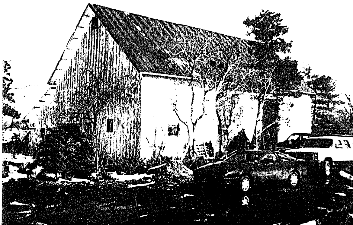
Figure 4.21 Framed barn (B. Roberts)
