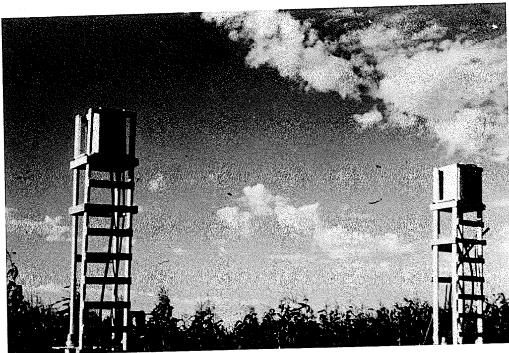
Figure 3.9 Towers and pressure regulating water reservoirs
