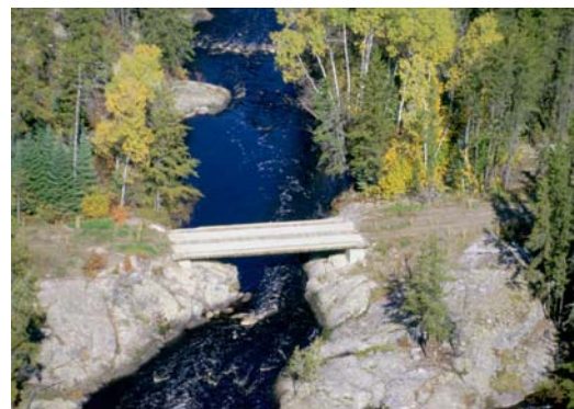
Removable bridge over the Black River constructed out of a recycled railway flatcar.
