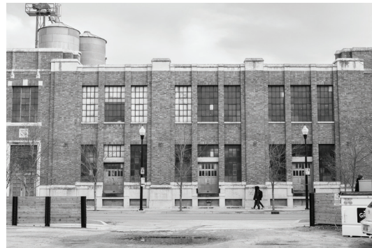
Figure 7.1 View of Building from Lily Street, by Katryna Lipinsky, 2021 [Photograph]
