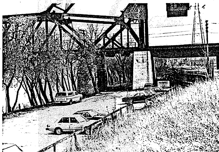
Figure 61. Parking on middle terrace and concrete pylons of CNR Bridge. Lombard North Group. Downtown Riverbank Park. Winnipeg: Lombard North Group, 1992.
