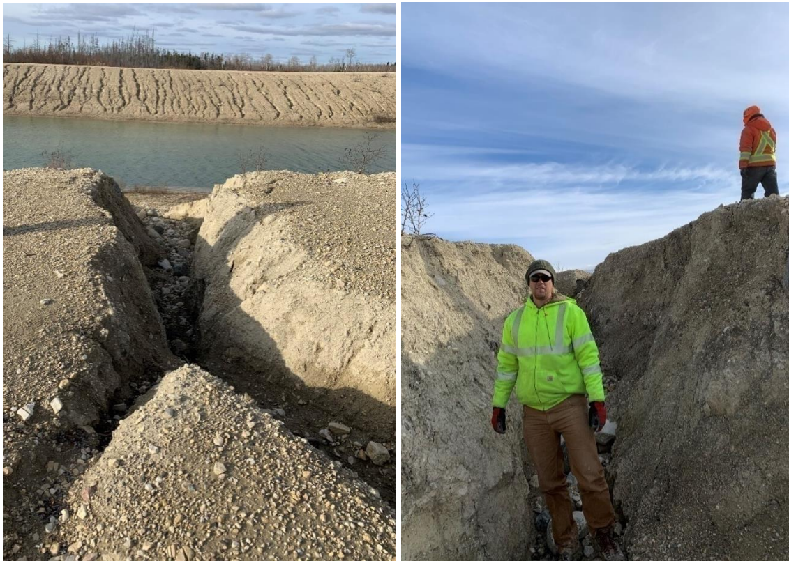
Figure 12: Rill erosion along banks of LSMEOC (person is 1.94 m tall)
