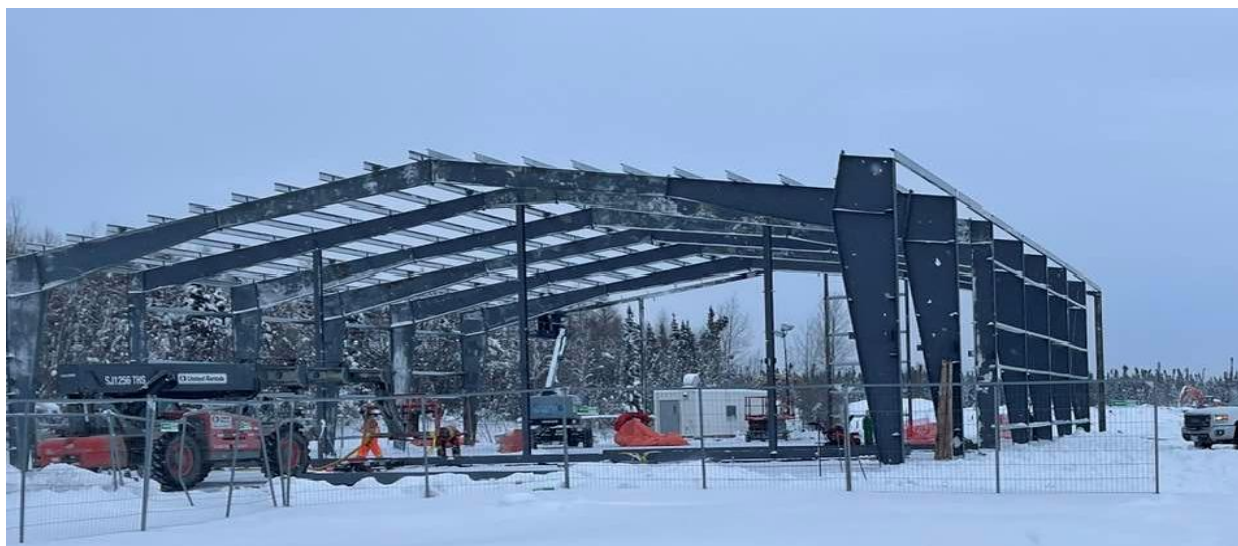
Figure 4.10: The Wikiwin Polytechnic Institute under Construction at York Landing in 2024
