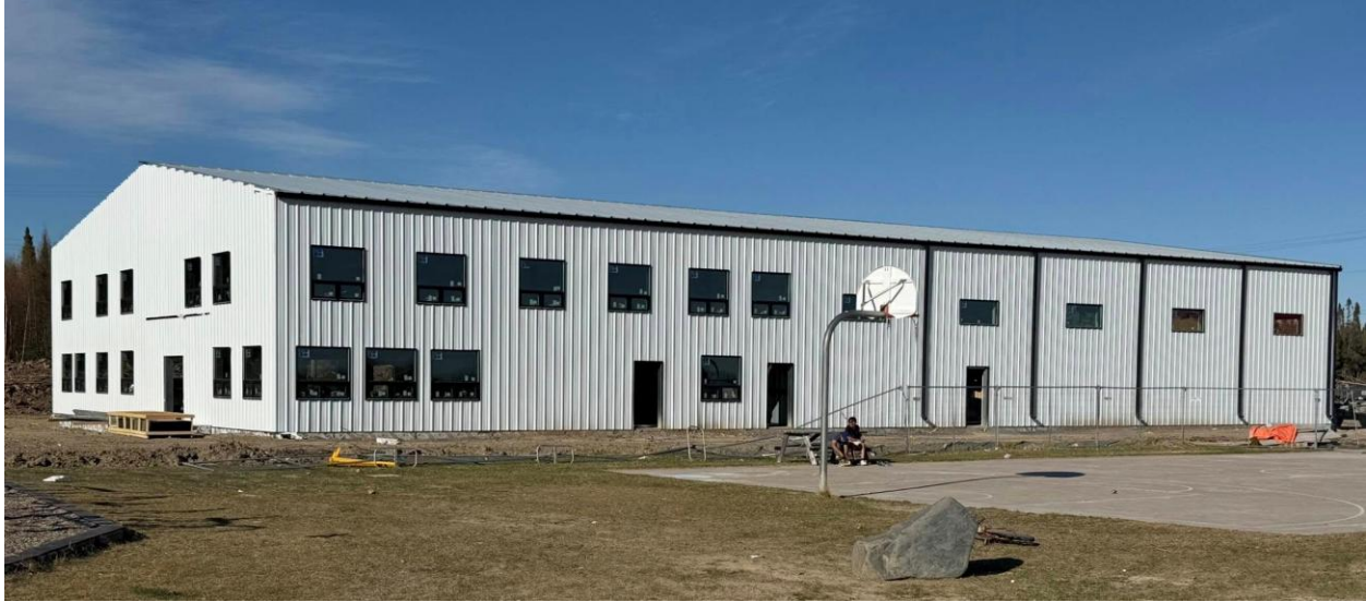
Figure 4.11: The Wikiwin Polytechnic Institute Shell completed at York Landing in 2025
