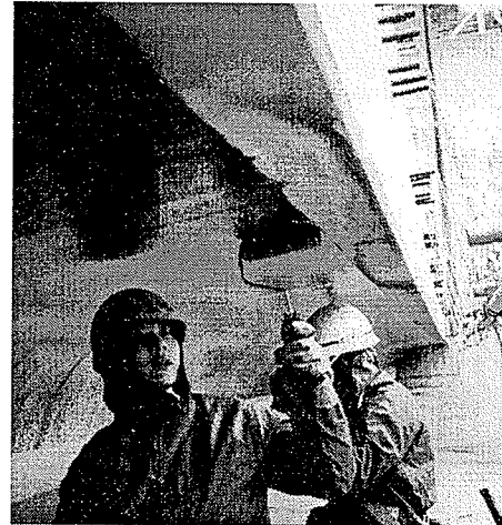
Fig. 2.34b Application of the resin coat [Nanni, 1995]
