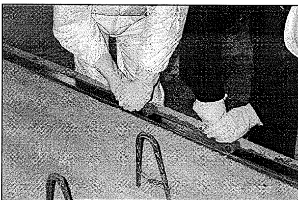
Fig. 3.16 Bonding the CFRP strips to the surface
