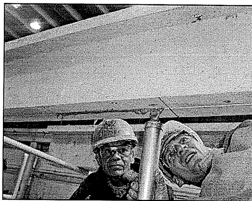
b) filling the groove with epoxy
