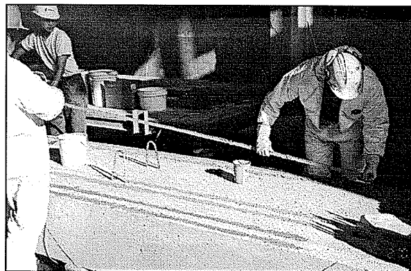
Fig. 3.19 Inserting the CFRP strips inside grooves
