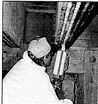
Fig. 2.30c Filling the grooves with epoxy [Gentile and Rizkalla, 1999]
