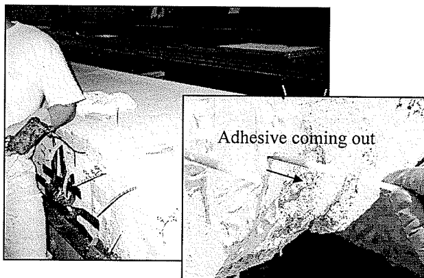
Fig. 3.13 Injecting the cracks
