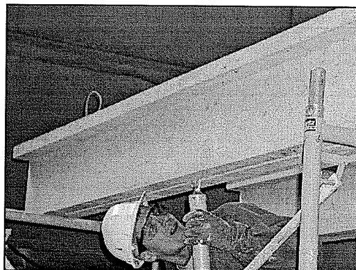
b) filling the groove with epoxy
