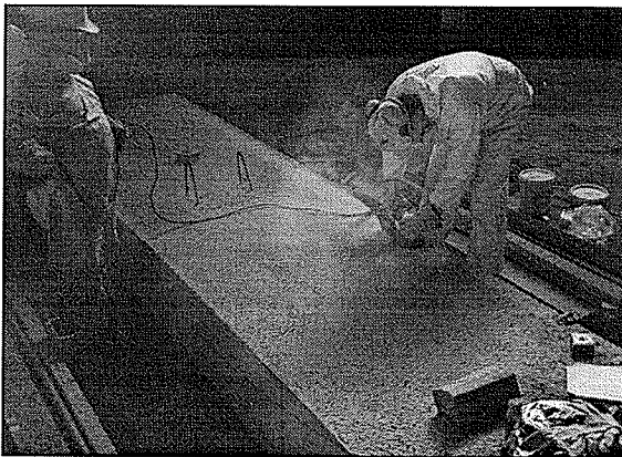
Fig. 3.14 Grinding the surface
