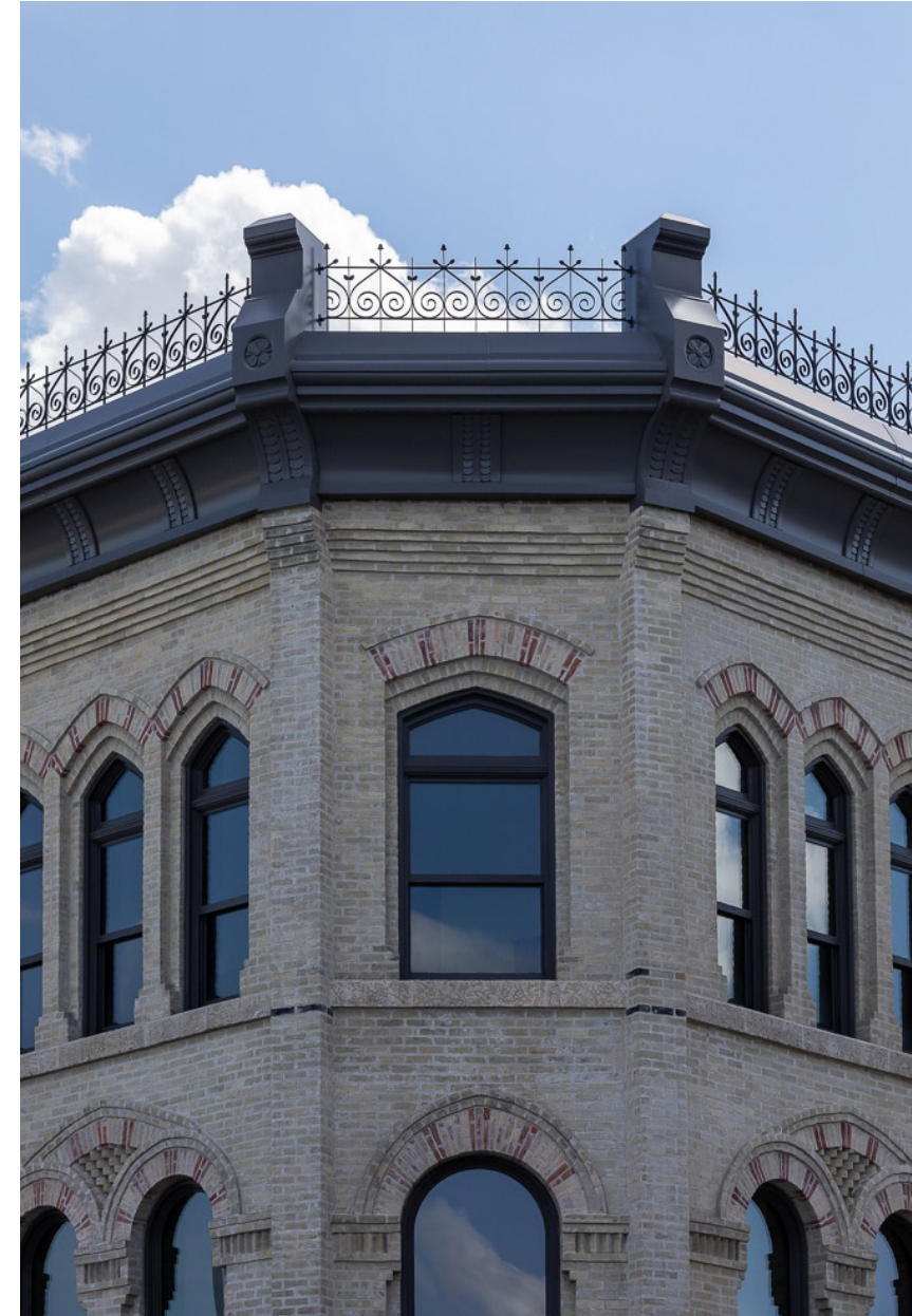
Fig 44: Cornice details, corbel and window details give it a unique building.
