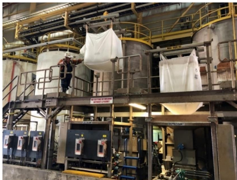
Figure 1: New bulk bag being installed using overhead crane and lifting device
