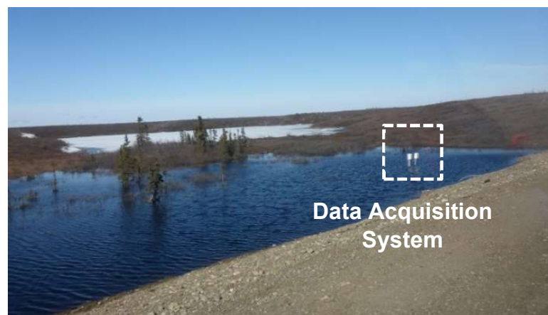
Fig. 3-3. Clogged upstream side of the culvert in May 2016.
