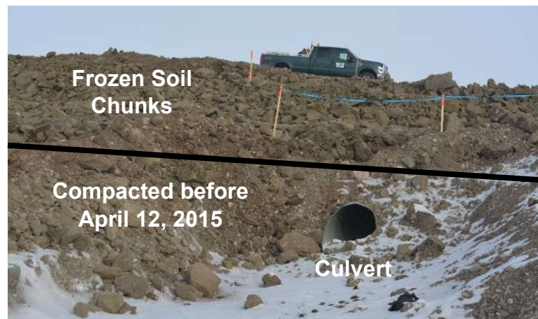
Fig. 3-2. Construction of highway fill embankment above the culvert at the research section of the University of Manitoba.
