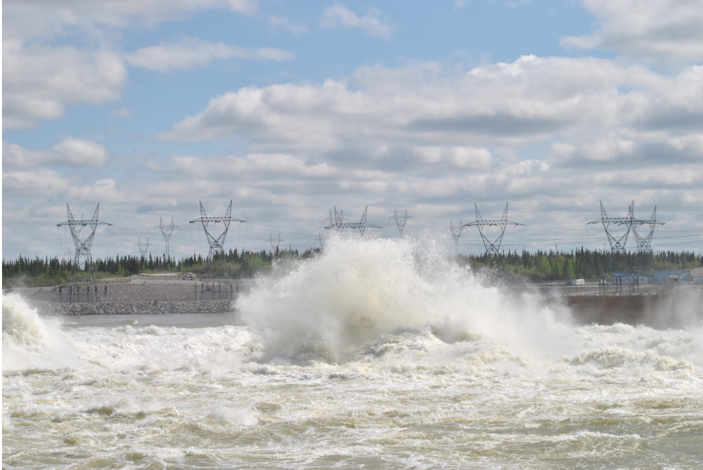
Figure 2. Limestone Generating Station near Gillam, Manitoba.
