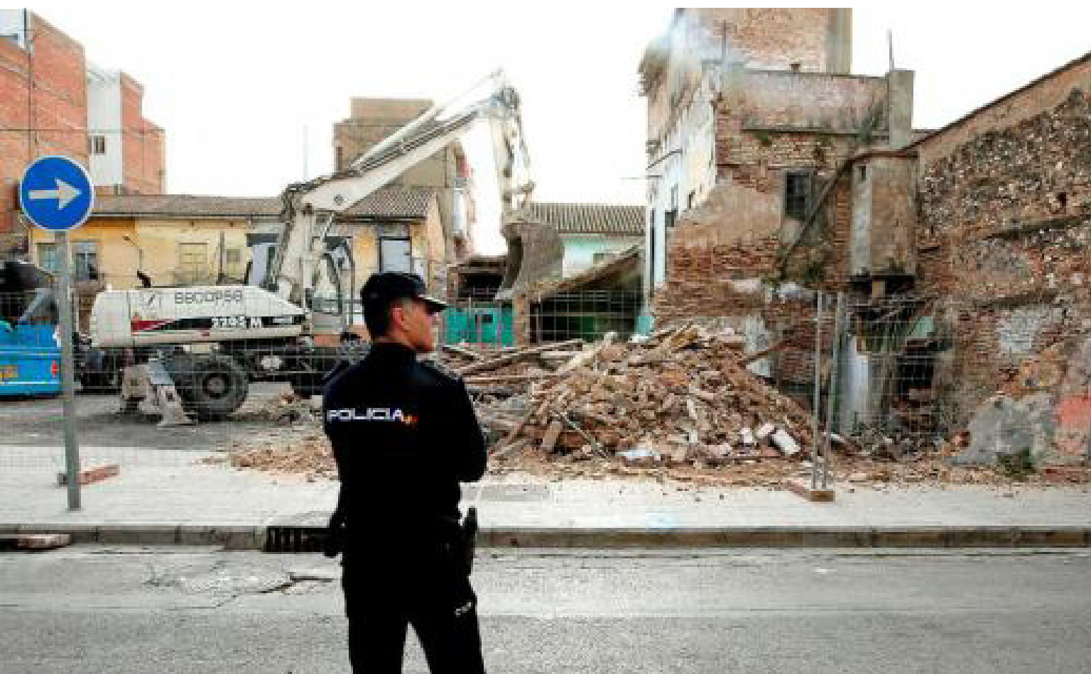
FIG.24. Police officer guarding the demolition of houses in El Cabanyal.
