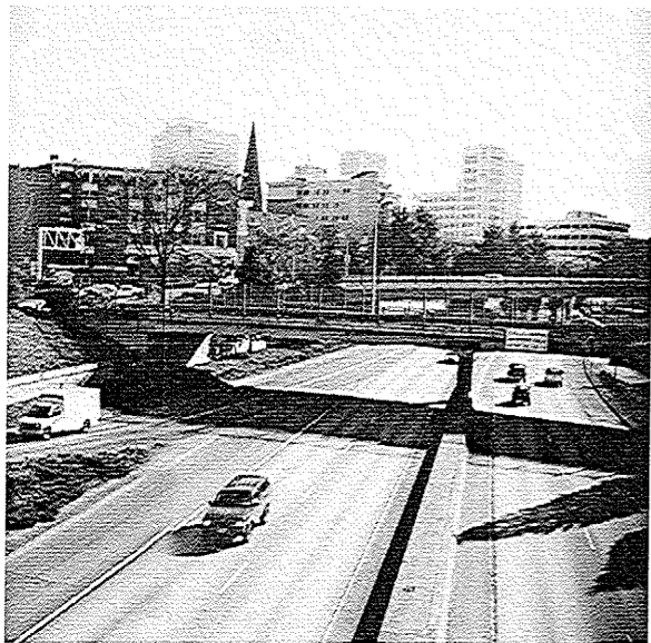
Figure 17. Site photo, Burnside and Alder bridges over I-405, taken from the Couch Street bridge.
