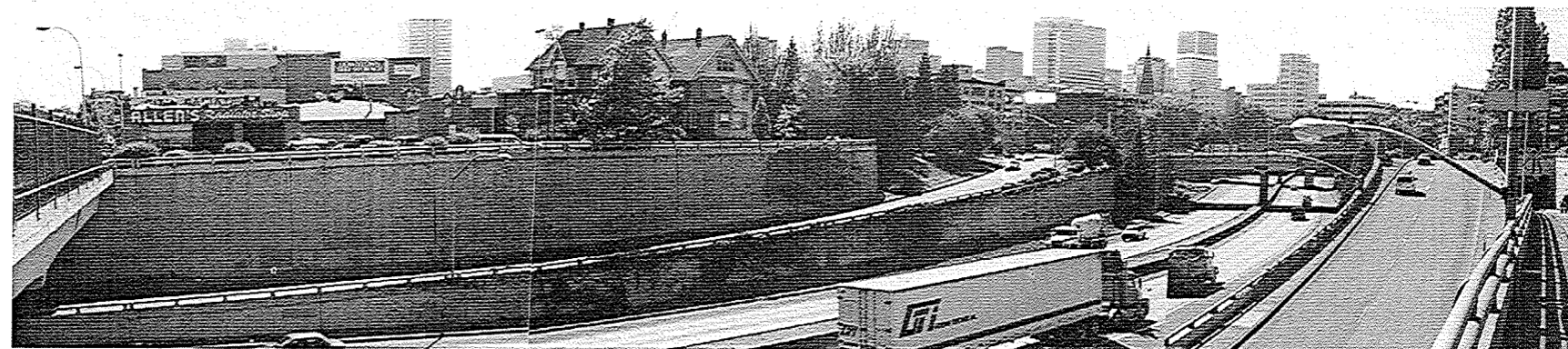
Figure 14. Looking south along I-405 toward downtown Portland, taken from 16th and Everett.
