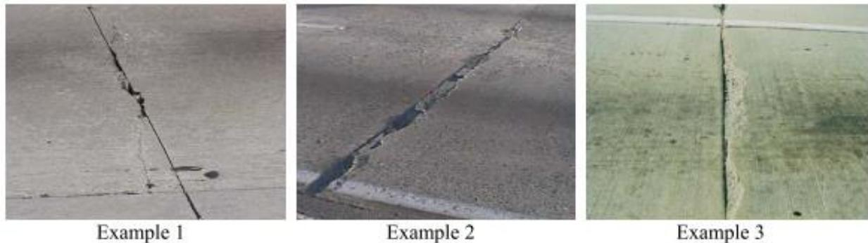
Figure 2-3: Examples of Joint Spalling (State of California Department of Transportation, 2004).
