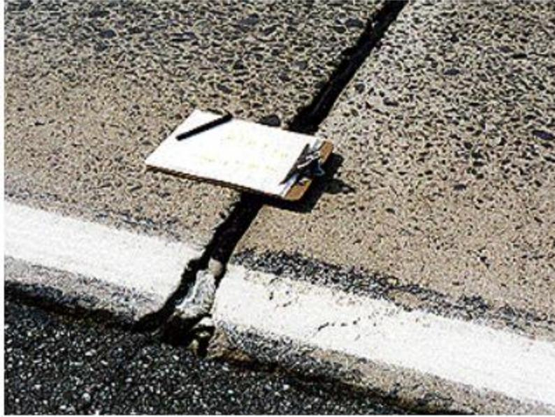
Figure 2-4: Joint Faulting (Federal Highway Administration, 2003).
