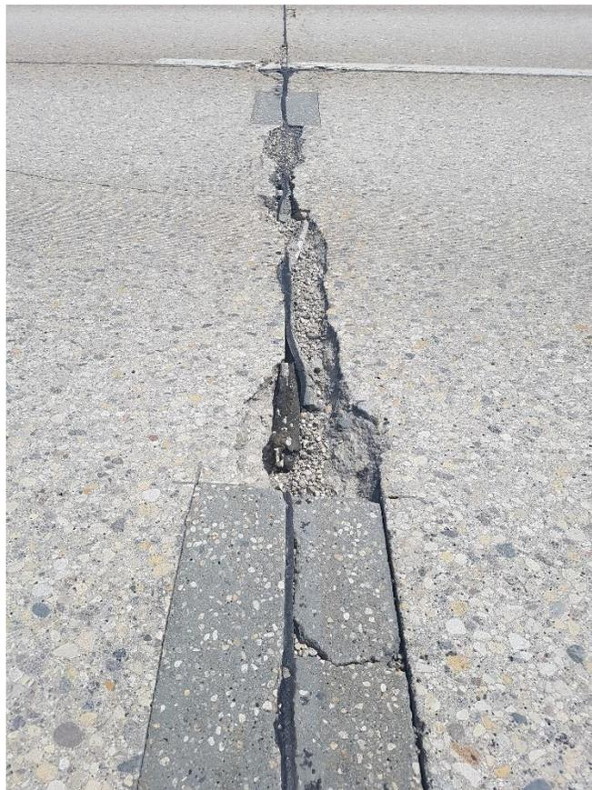
Figure 2-12: Severely Cracked and Deteriorated Joint.
