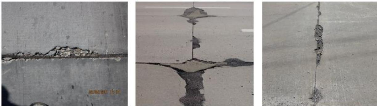
Figure 2-1: Typical Joint Deterioration (Wang et al., 2018).
