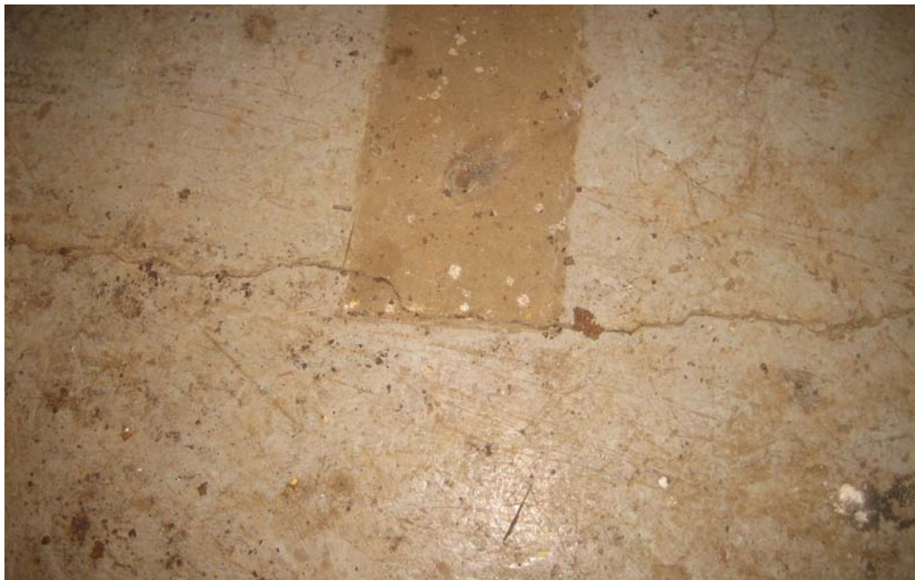
Cracked slab
