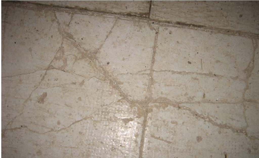
Cracked slab
