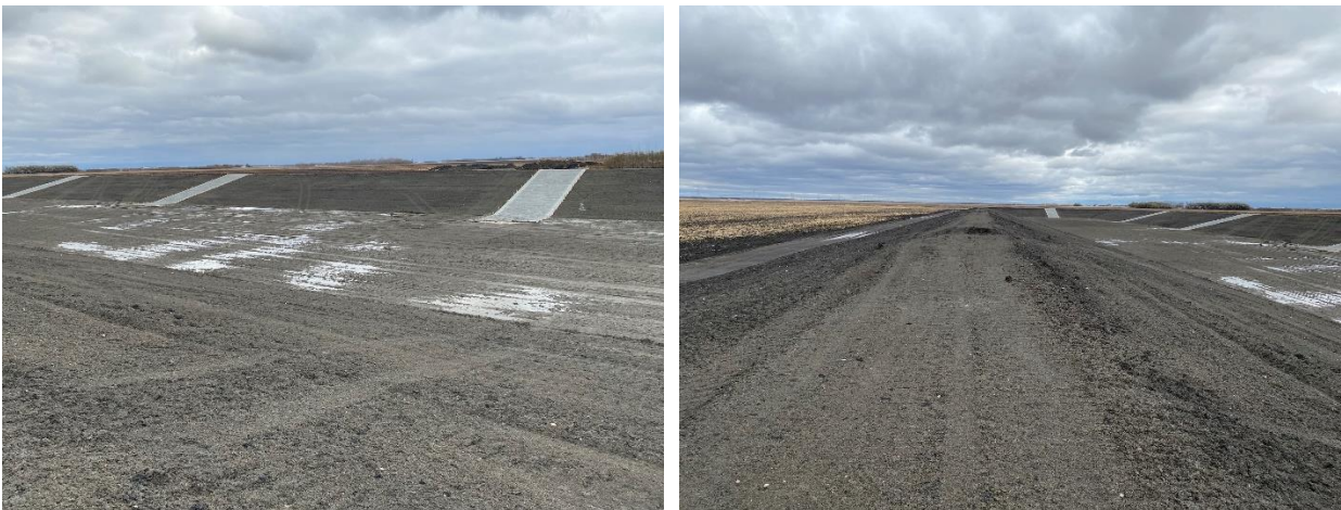
Figure 5 - Photos of EMS Floor (left) and Berm (right)
