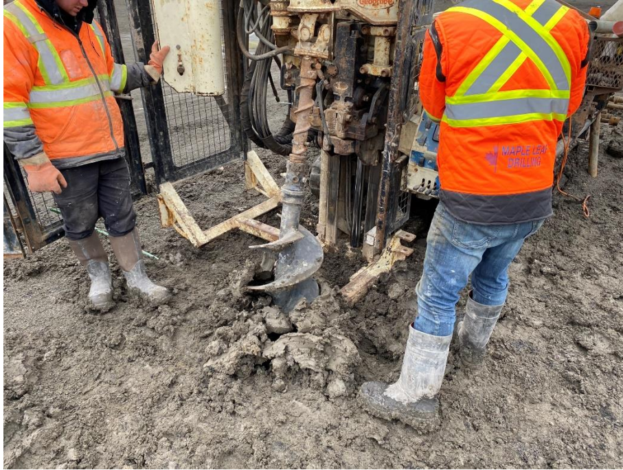
Figure 6 - Drilling of Borehole Infiltration Chamber
