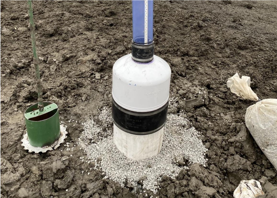
Figure 7 - Installation of Apparatus
