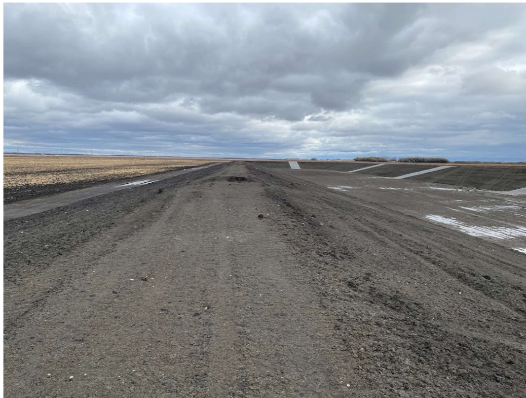
Picture 2: Site view of berm looking east
