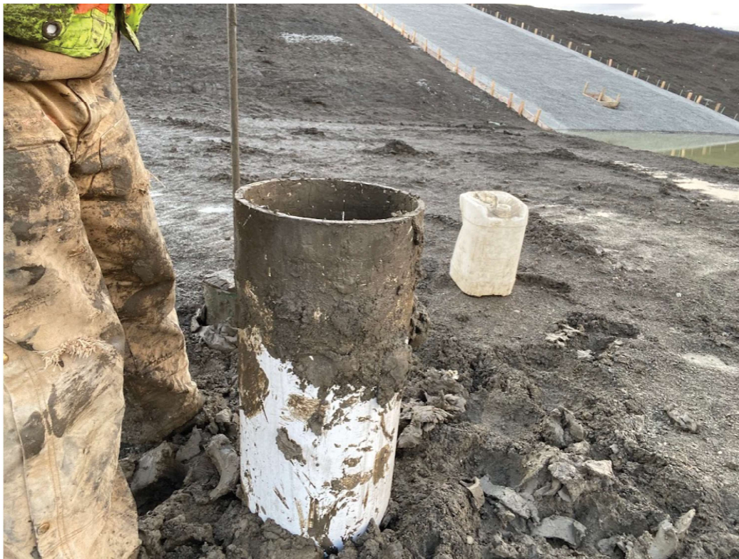
Picture 6: Advancement of stage 2 of berm test
