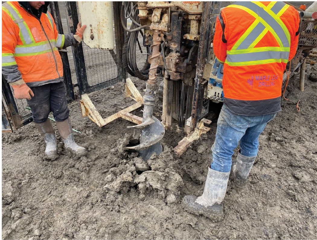
Picture 3: Drilling borehole for berm test
