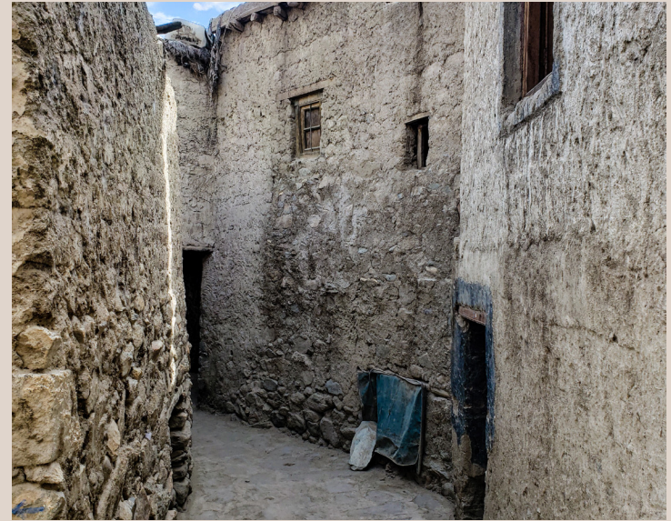
(B) Figure 40: Some parts of Kharyog still display the heritage of Leh and are relatively untouched by modern construction techniques. The street above lies in such an area and shows the narrow streets without any drainage infrastructure.
