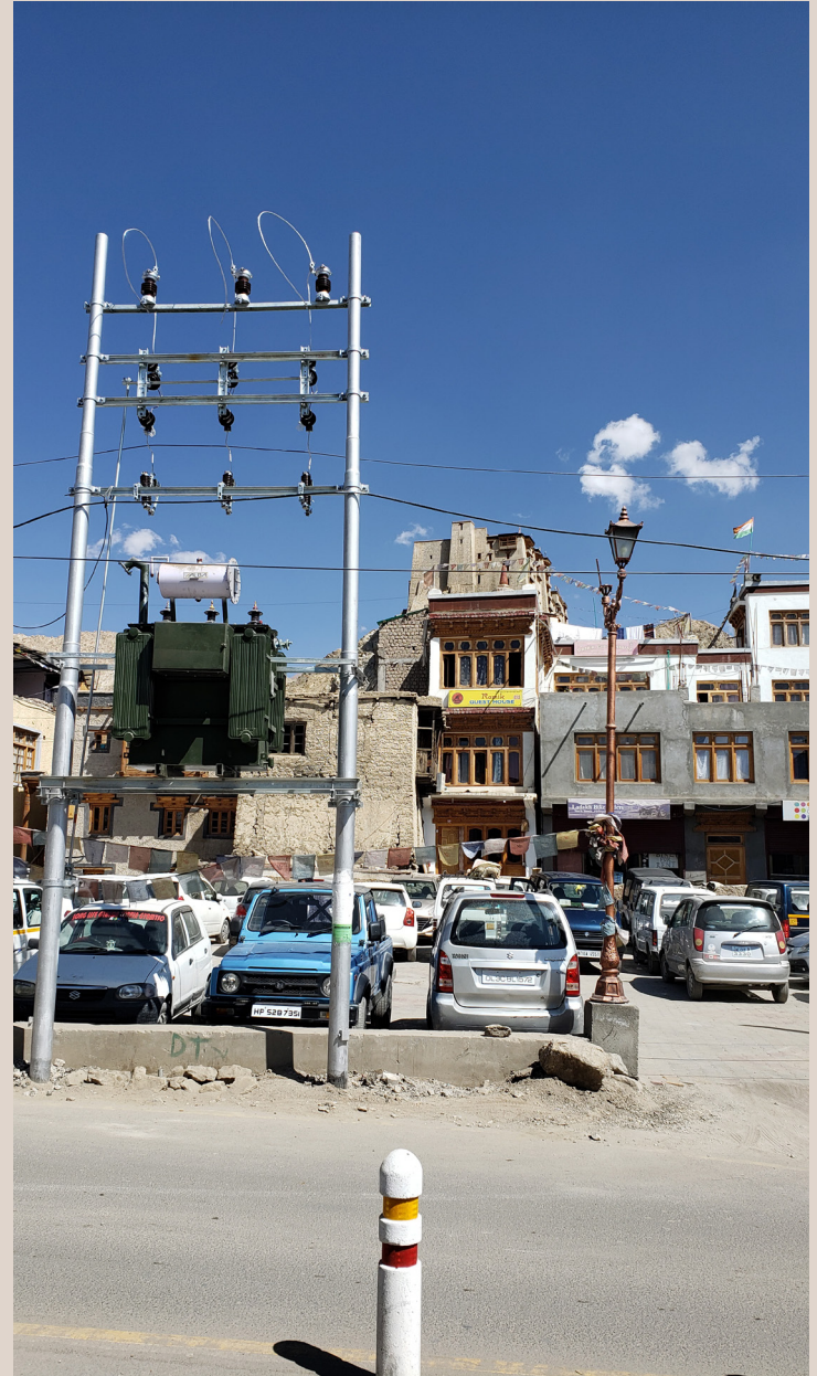
G Figure 73: The east side of Old Fort Road is missing a sidewalk. Adjacent to its intersection with Chutey Rantak street is a car park.
